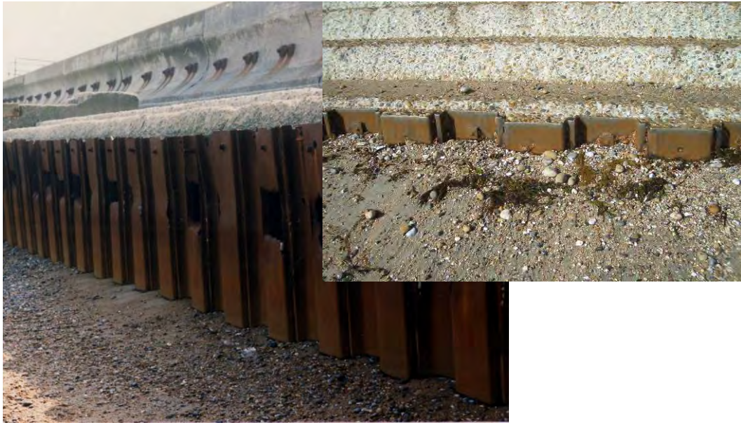
Figure 2.2 Sheet pile underpinning
