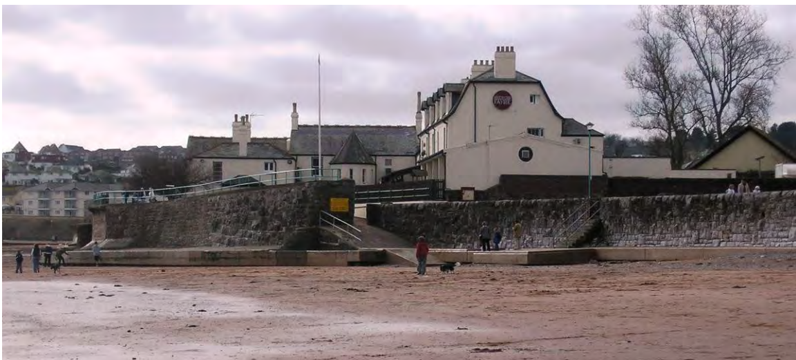
Figure 5.22 Toe apron proves walking platform – Paignton, Devon (courtesy of ENBE)
