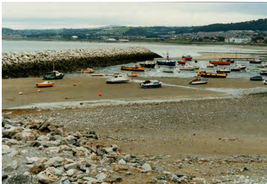
Figure C13.2 View to the east showing usage by small boats
