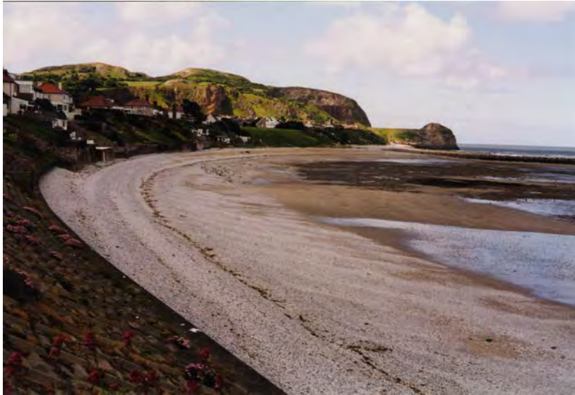
Figure C14.3 View of beach recharge in western part of Penrhyn Bay
