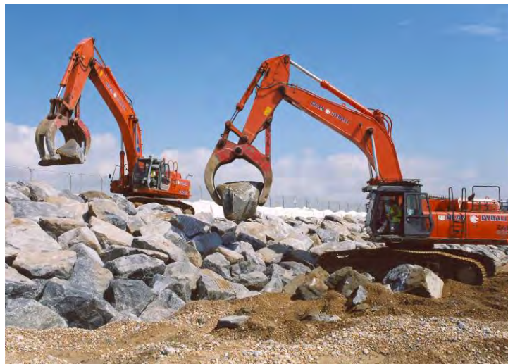
Figure 4.14 Manoeuvring armourstone blocks in a revetment (courtesy Dean and Dyball Ltd)
