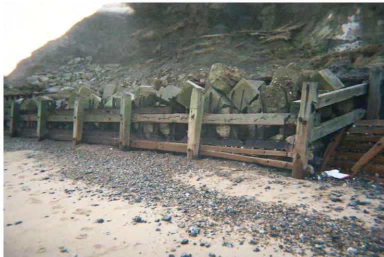
Figure 2.3 Cribwork and concrete block fill, Norfolk (courtesy of North Norfolk District Council)
