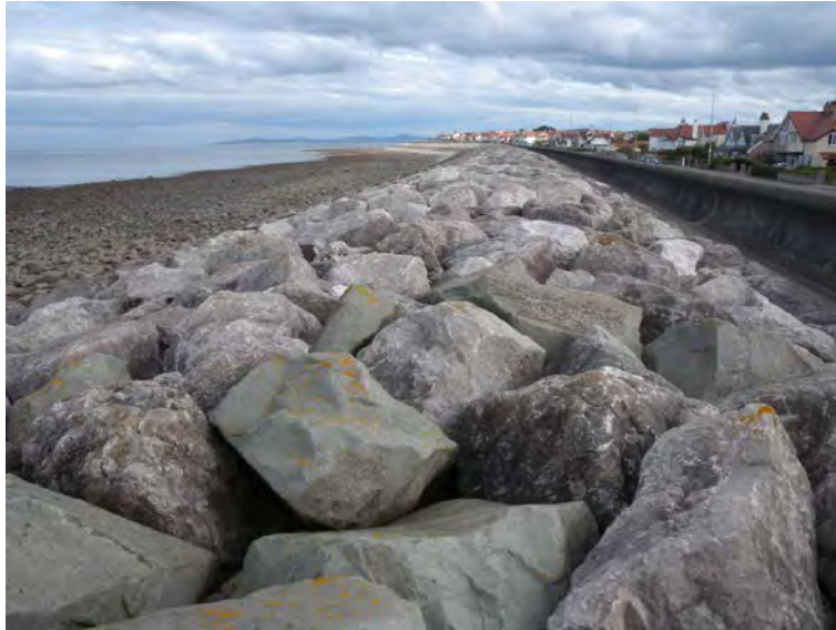
Figure C14.5 View along rock revetment protected frontage to east (CEUK)
