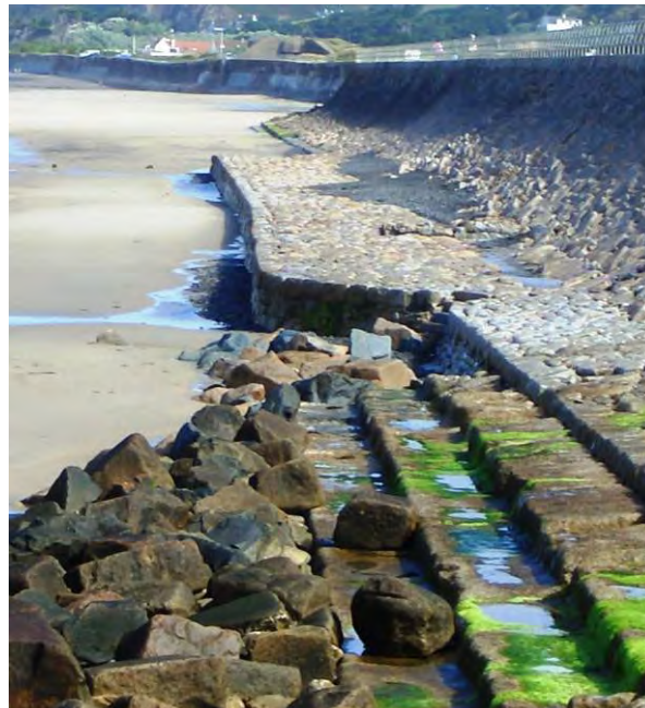
Figure 2.8 Extended scour apron, masonry steps and armour, St Ouens Bay, Jersey (courtesy HR Wallingford)
