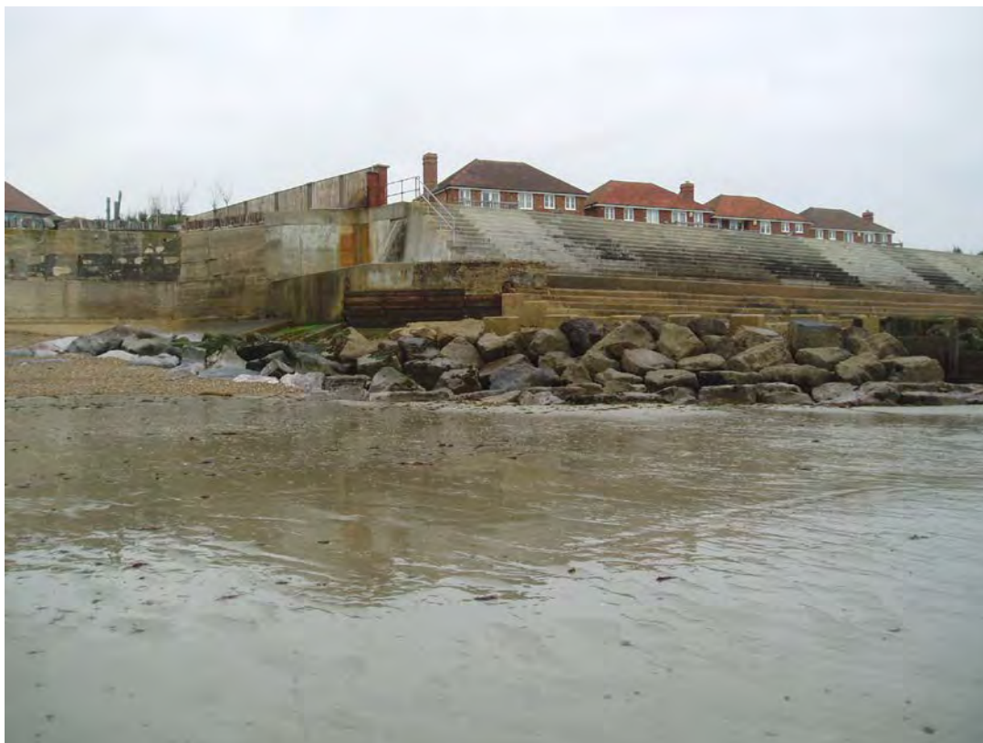
Figure C9.4 The completed armour revetment
