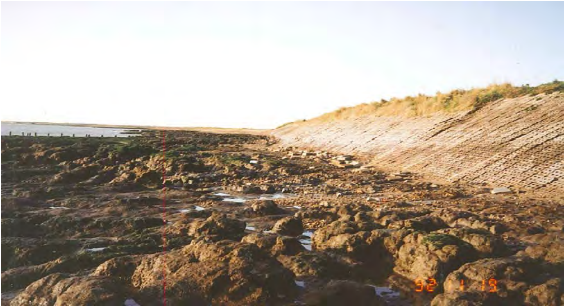
Figure C6.2 Flexible armoured revetment (earlier defence structure)
