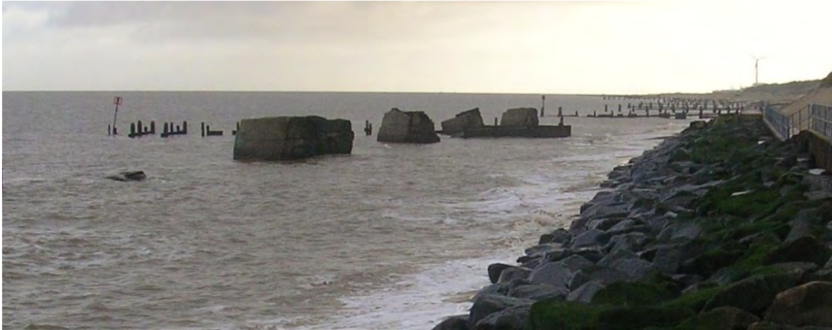
Figure C2.2 Detached concrete relics of 1870 Colman coast defences
