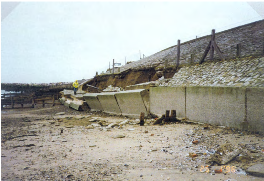
Figure C10.3 Failure damage, 1996
