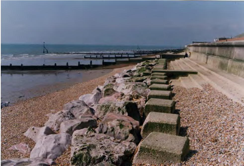
Figure C17.2 Toe berm of rock and concrete armour units, 1994
