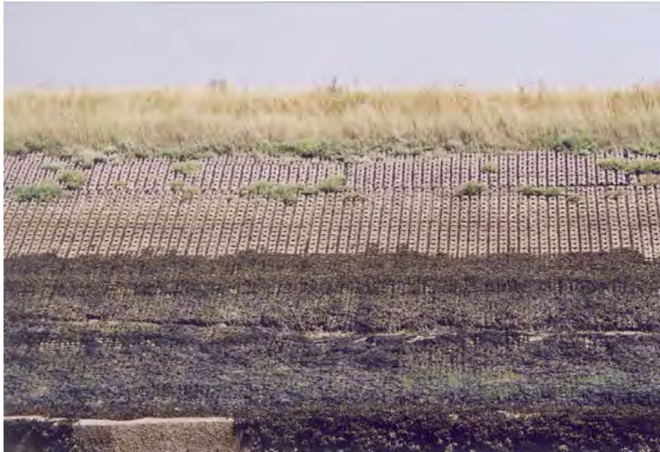
Figure 5.19 Example of a flexible armoured revetment
