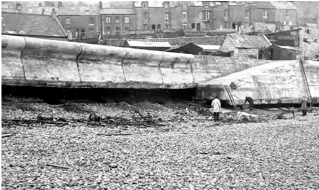
Figure 4.9 Unsupported section of reinforced mass concrete seawall following major undermining (Chesil Cove 1962) © Stuart Morris
