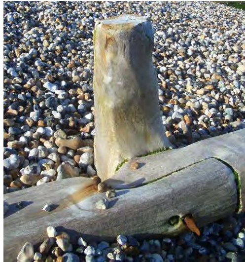
Figure 2.21 Rounding of groyne timbers by beach shingle (courtesy HR Wallingford)
