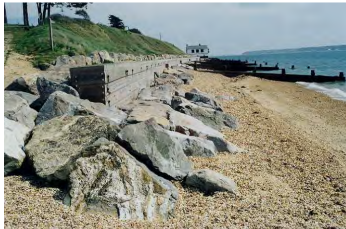
Figure 2.7 Timber bulkhead with rock toe protection at Lepe, Hampshire
