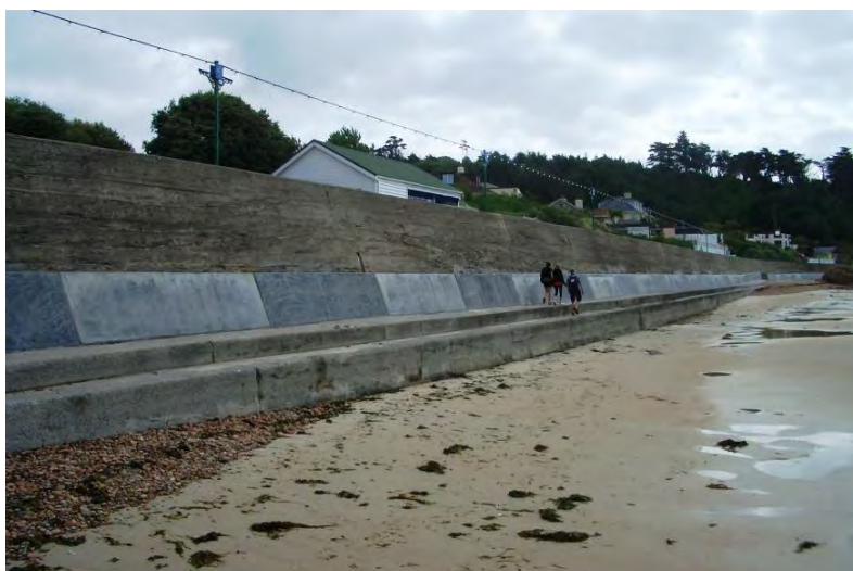
Figure 2.14 Concrete toe beams (courtesy HR Wallingford)
