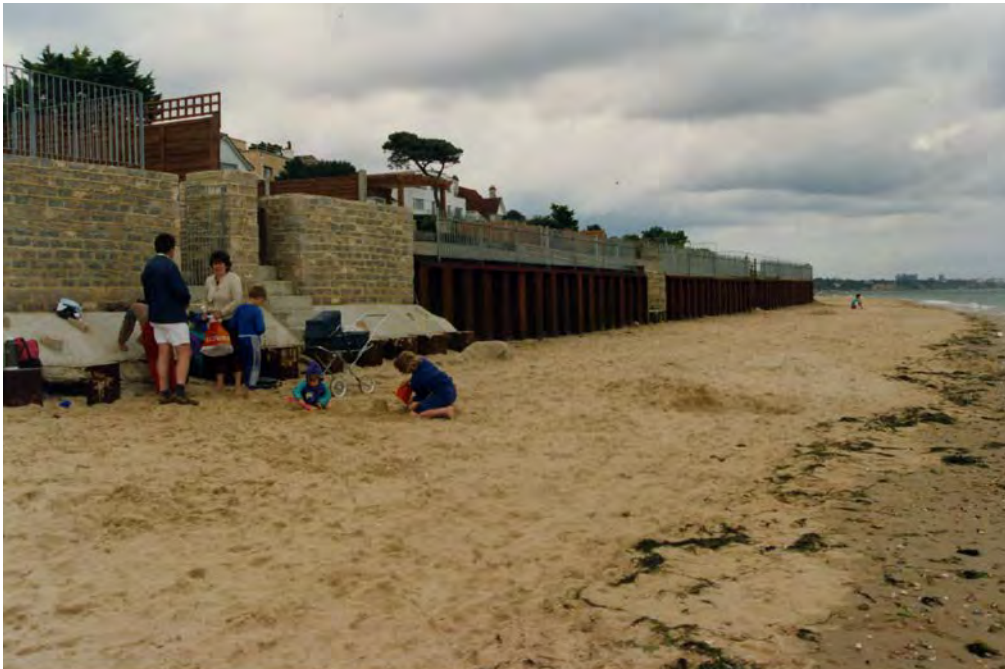
Figure C15.1 Vertical wall and low beach near Haven Hotel, Sandbanks, c.1998
