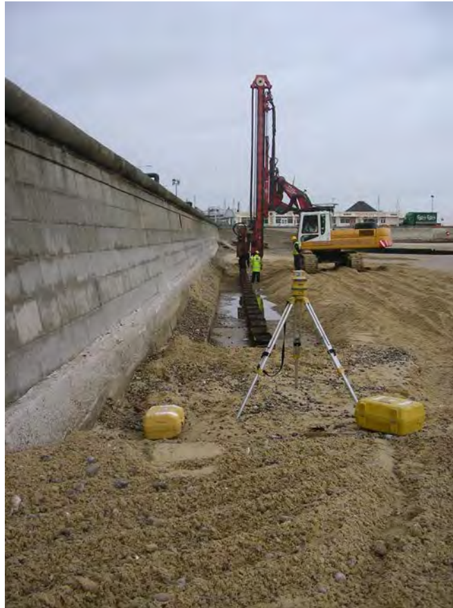
Figure C3.6 Toe piling being installed (at concrete wall section)
