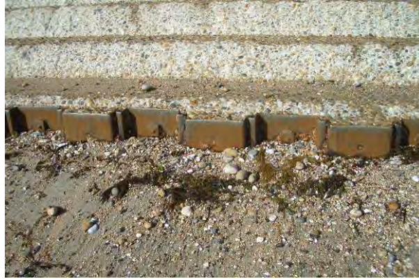
Figure 2.1 Underpinning of seawall toe with steel sheet piles (courtesy HR Wallingford)
