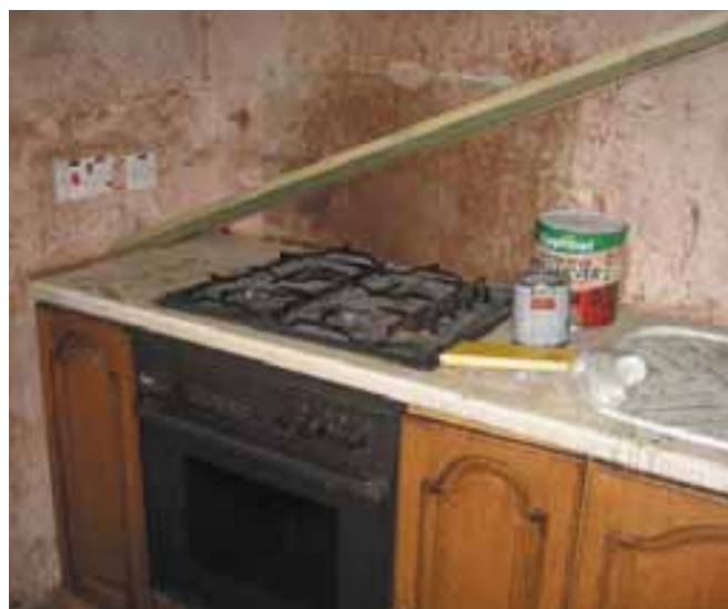
Figure 1: surface swab sampling in the kitchen © HPA
