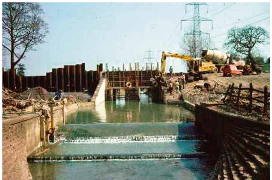
↑ Construction work at Tubbs Bottom
