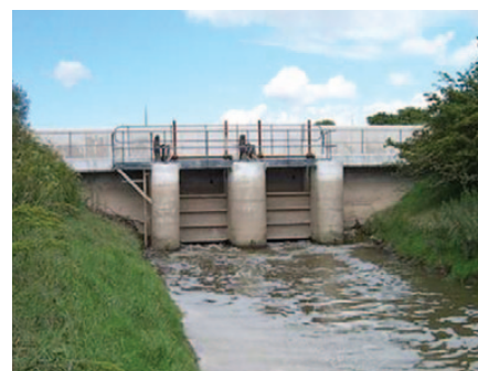
↑ Tidal Outfall on Main Dyke
