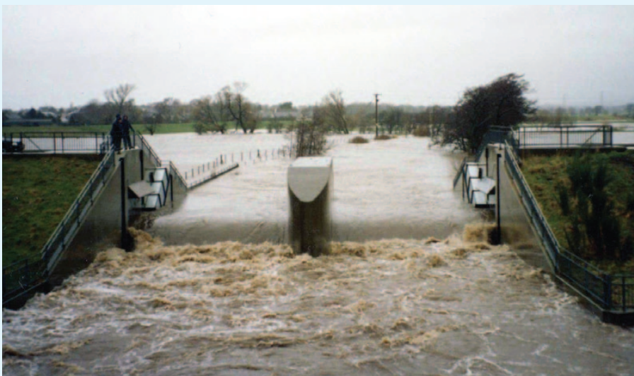
↑ Garstang Flood Basin in operation
