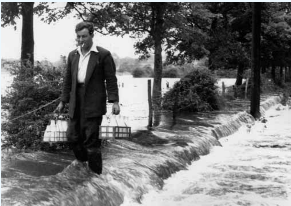
↑ A milkman walks along a wall top through floods from the River Frome at Lower Burton July 1955
