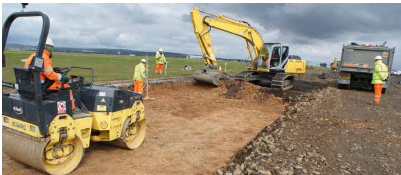
Reusing the aggregate prior to resurfacing © Lend Lease/Debut
