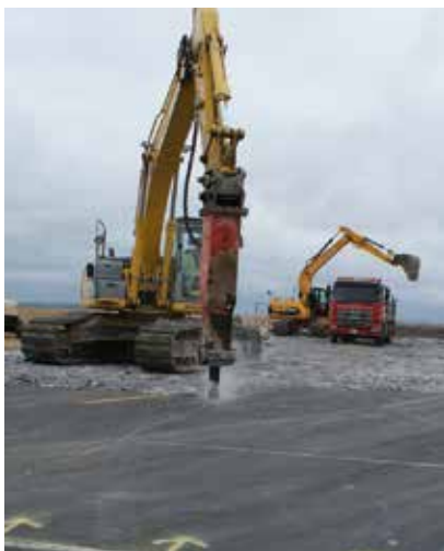
Breaking the concrete © Lend Lease/Debut
