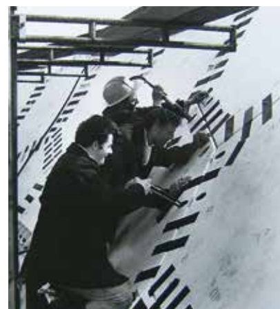
30th May 1962: Construction workers fitting Radome panels © RAF Fylingdales/Crown
