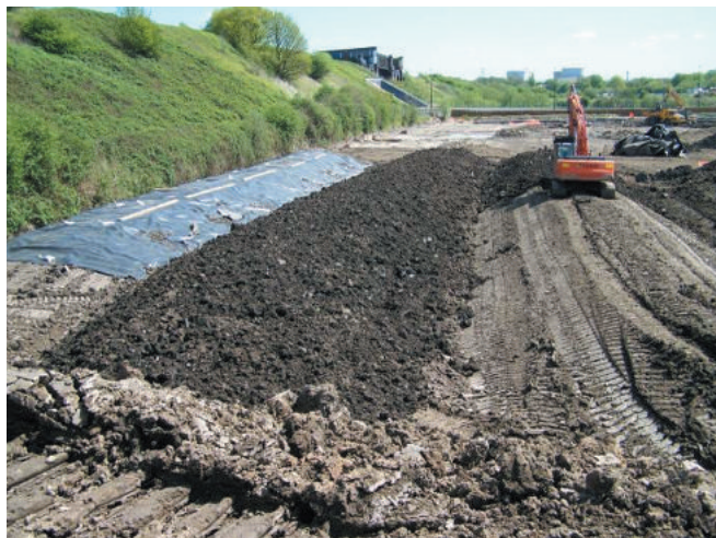
Figure 4: Windrow covering and aeration (Source: Steve Edgar, Vertase FLI Ltd)
