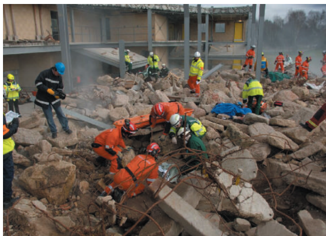
Figure 4: Exercise Orpheus – Urban Search and Rescue teams work through the rubble from an unstable collapsed multi-story building (Image © HPA, 2008)
