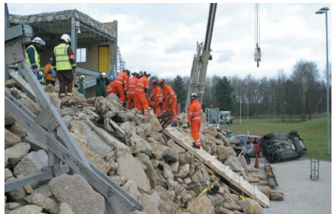
Figure 2: Exercise Orpheus - Urban Search and Rescue teams work in an unstable collapsed multi-story building (Image © HPA, 2008)
