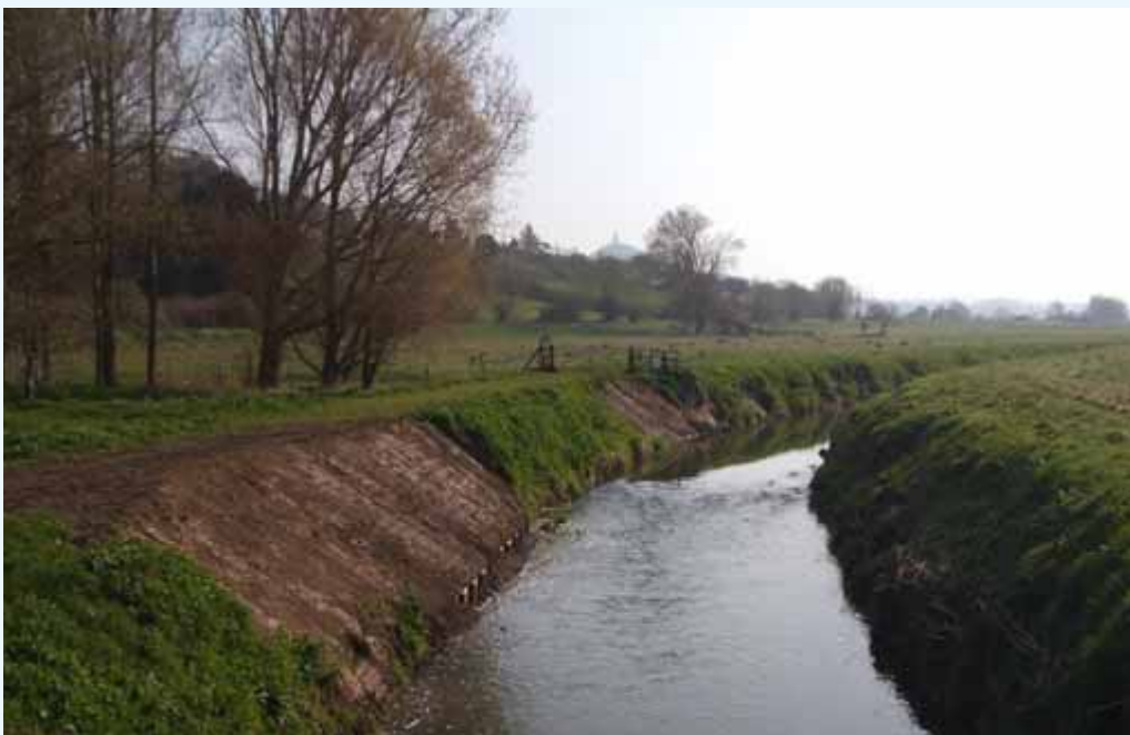
↑ Minor works undertaken on the River Brue near Glastonbury
