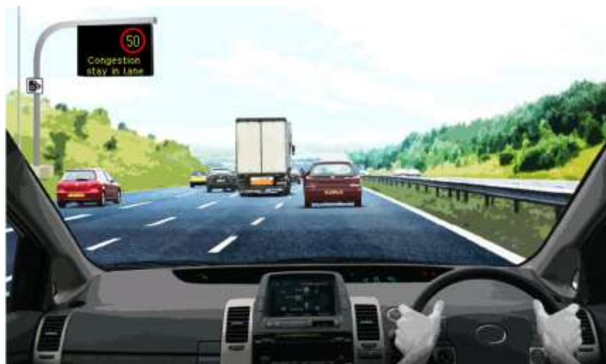
Figure 4D: Illustrative M5 Junction 4A to 6 Smart Motorway All lane Running scheme section operating with variable mandatory speed limits and information for road users.
