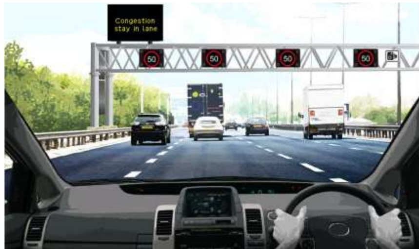
Figure 4C: Illustrative M5 Junction 4A to 6 Smart Motorway All lane Running scheme section operating with variable mandatory speed limits
