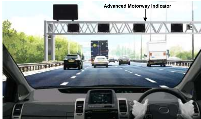
Figure 4A: Illustrative M5 Junction 4A to 6 Smart Motorway All lane Running scheme section operating in normal motorway conditions with blank advanced motorway indicators and blank gantry mounted variable message sign
