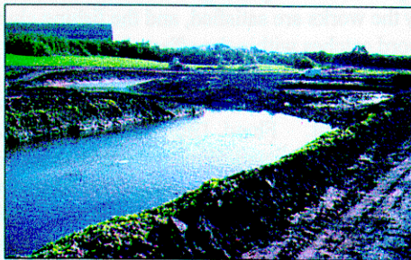
Meanders being constructed
