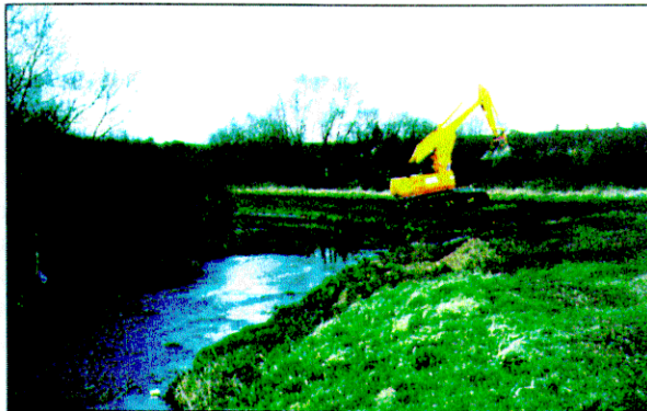
2c Steel piling being removed
