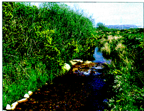
View of River Fal showing completed weir
