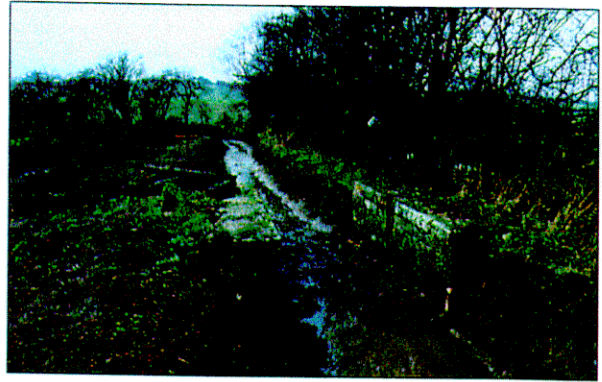
Feed system and sluice restoration
