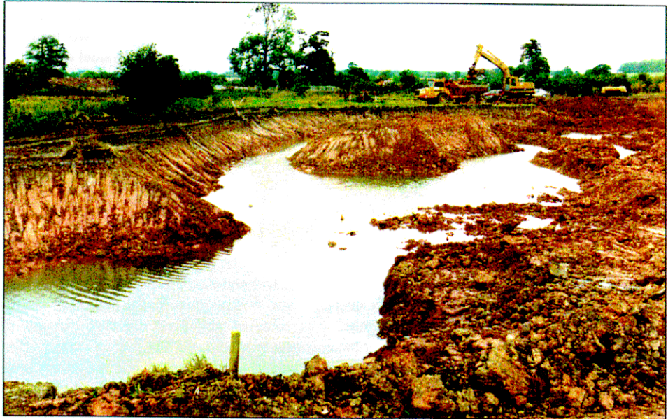
Lake construction showing varied slopes, depths and island
