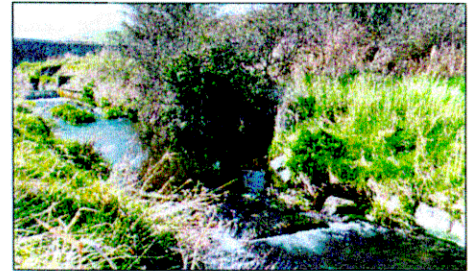
C1 – One of six boulder weirs raising water levels in fen
