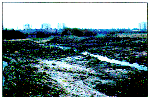
Cross-section 'C' during construction
