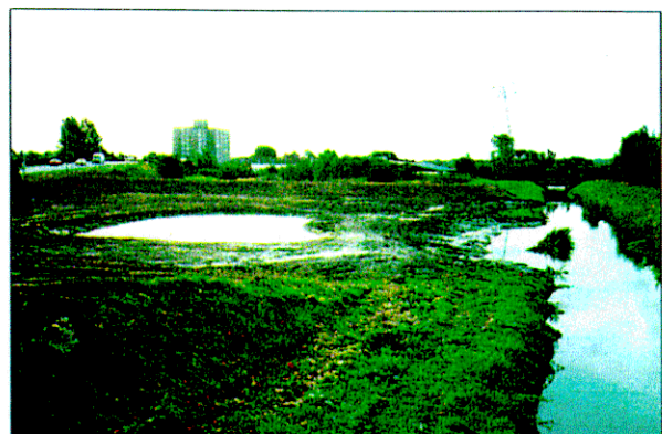
Reach 3 – Pond formed, planting and channel rehabilitation awaiting
