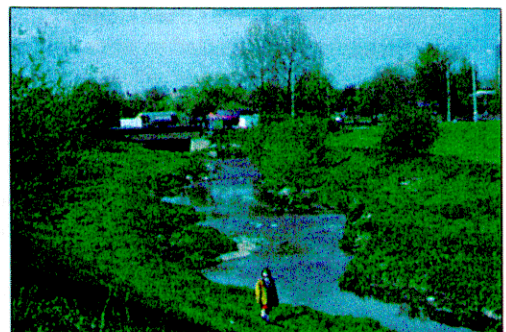
4 Riffle on Cole established on former weir
