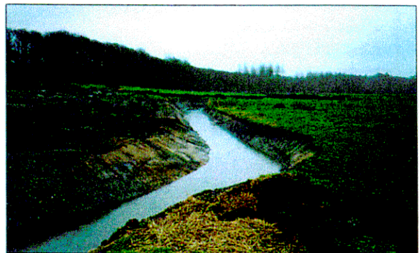
B – Channel dug in open field
