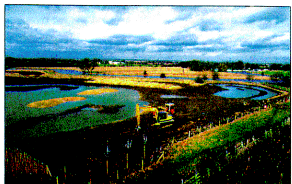
2 Main pond, pool and reedbed creation (February 1992)
