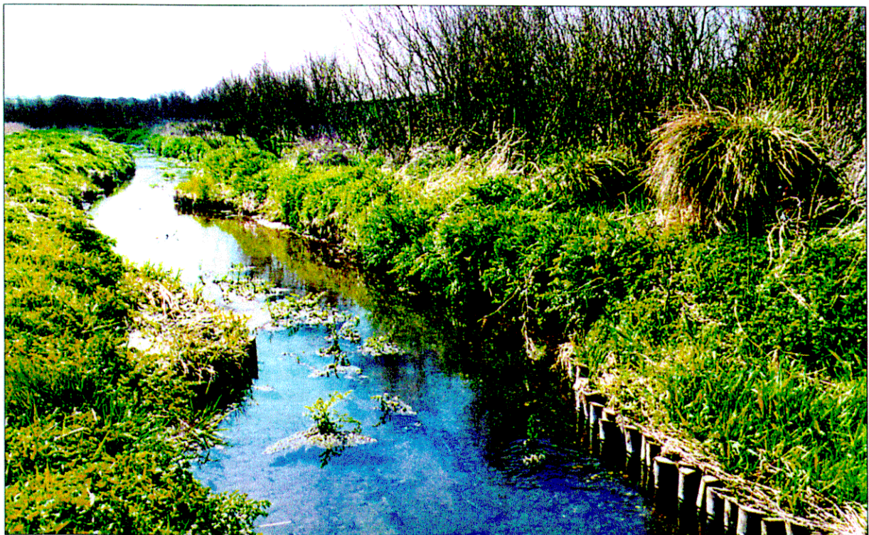
B – 'Meandering' of straight channel using pole revetment and reed infill
