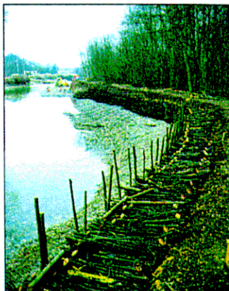
Oak Weir—River bank during work (Nov 1993–March 1994)
