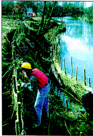
3 Branbridges—Installing Spilling Revetments (March 1994)
