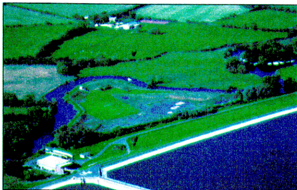
3 Aerial view of site – 3 years after (October 1995)
