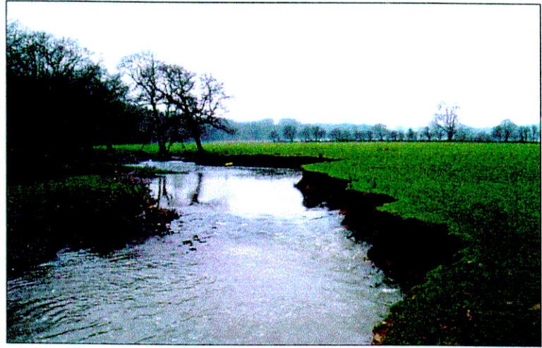
Tree removal, followed by loss of riparian vegetation through over-grazing causes erosion
