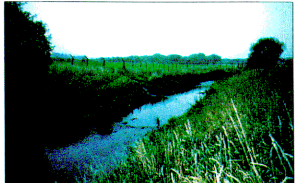
2b Steel piling of 2a masked by earth and vegetation
