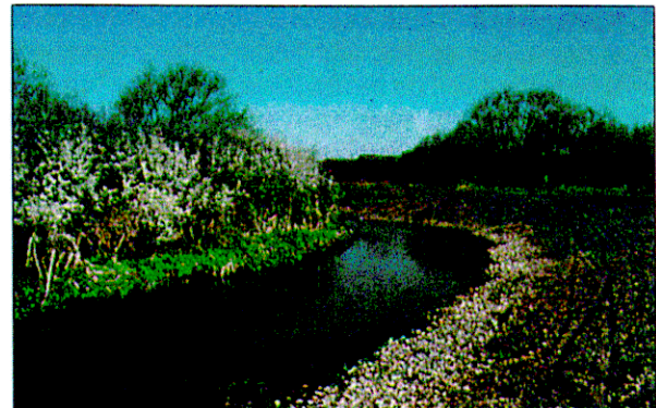
2d Steel piles of 2c removed and earth / stone bank in place
