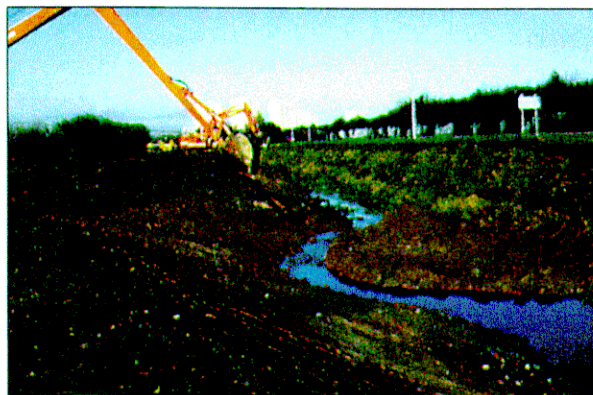
Cross-section 'B' being constructed
