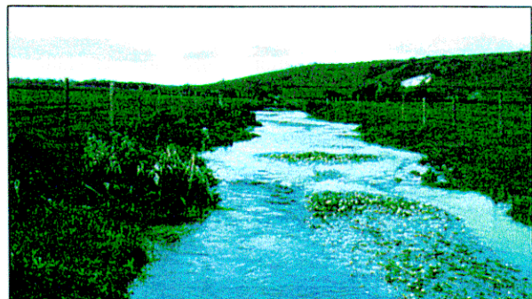
4 After instalation of groynes
