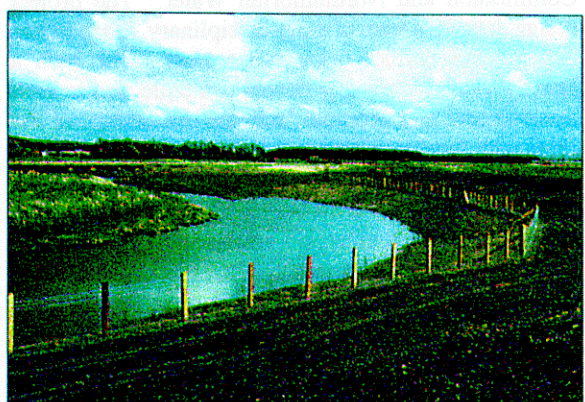
Cut-off meander restored, banks re-seeded and fenced
