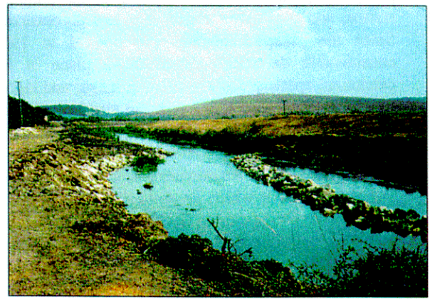
Work in progress – Summer 1995
