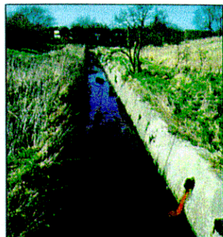
3a Yardley Brook – Concrete channel upstream of 3b
