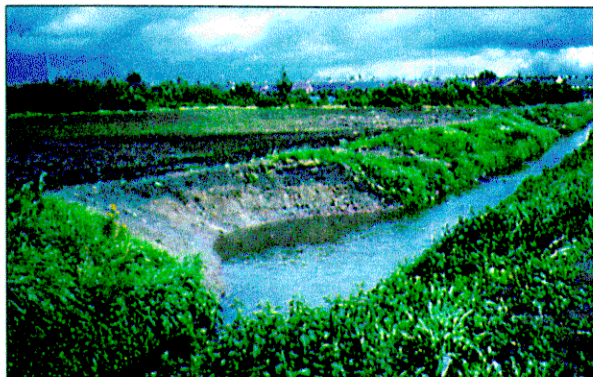
Channel prior to scheme showing uniform banks with bays constructed in 1993
