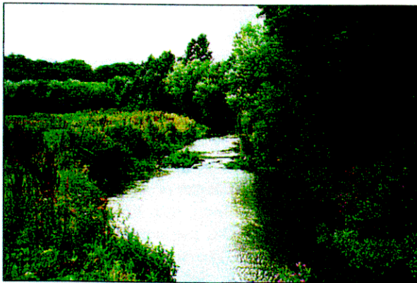
Weir on Stiffkey
