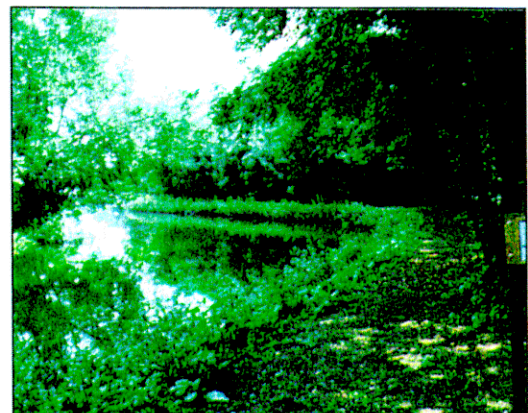
Oak Weir—View of bank after completion of work (June 1994)
