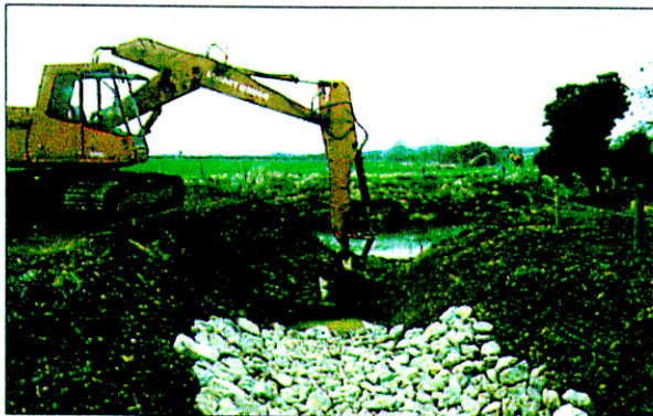
A Re-opening of meander showing stone armouring – (1992)
