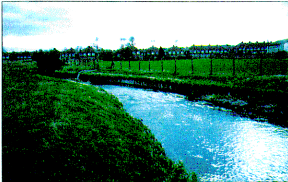
2a Steel piling prior to masking
