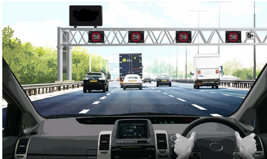
Figure 4C: Illustrative M25MM section operating with Variable Mandatory Speed Limits
