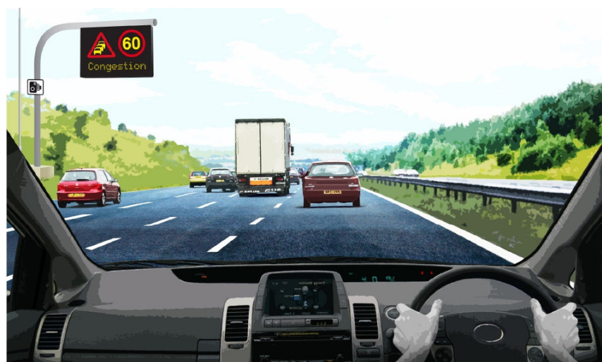
Figure 4D: Illustrative M25MM section operating with Variable Mandatory Speed Limits and information for road users
