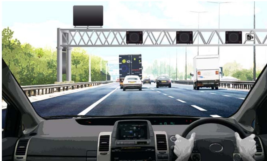
Figure 4.2A: Illustrative M60 J8 to J18 controlled motorway section of the smart motorway scheme section operating in normal motorway conditions with blank advanced motorway indicators and blank gantry mounted variable message sign
