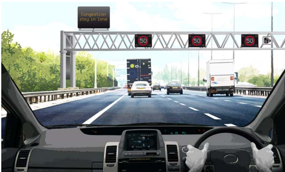
Figure 4.3A Illustrative M60 J8 to 18 controlled motorway section of the smart motorway scheme operating with variable mandatory speed limits
