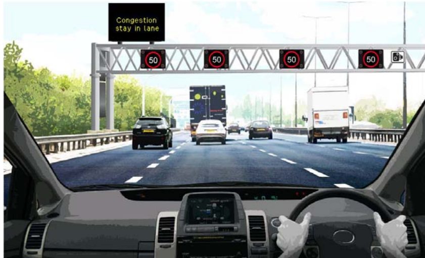
Figure 4.3C: Illustrative M62 J18 to J20 smart motorway scheme section operating with variable mandatory speed limits
