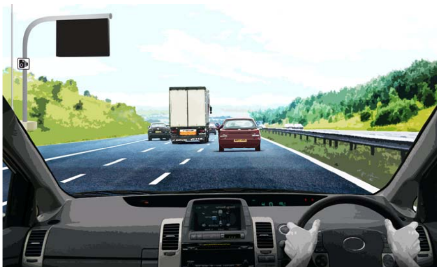
Figure 4.2B: Illustrative M60 J8 to J18 controlled motorway section of the smart motorway scheme section operating in normal motorway conditions with a blank verge mounted variable message sign
