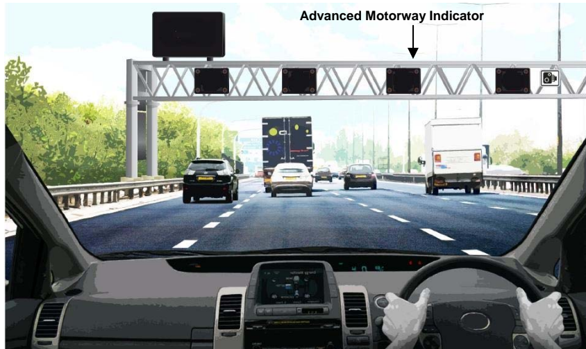
Figure 4.2C: Illustrative M62 J18 to J20 of the smart motorway all lane running section of the smart motorway scheme operating in normal motorway conditions with blank advanced motorway indicators and blank gantry mounted variable message sign
