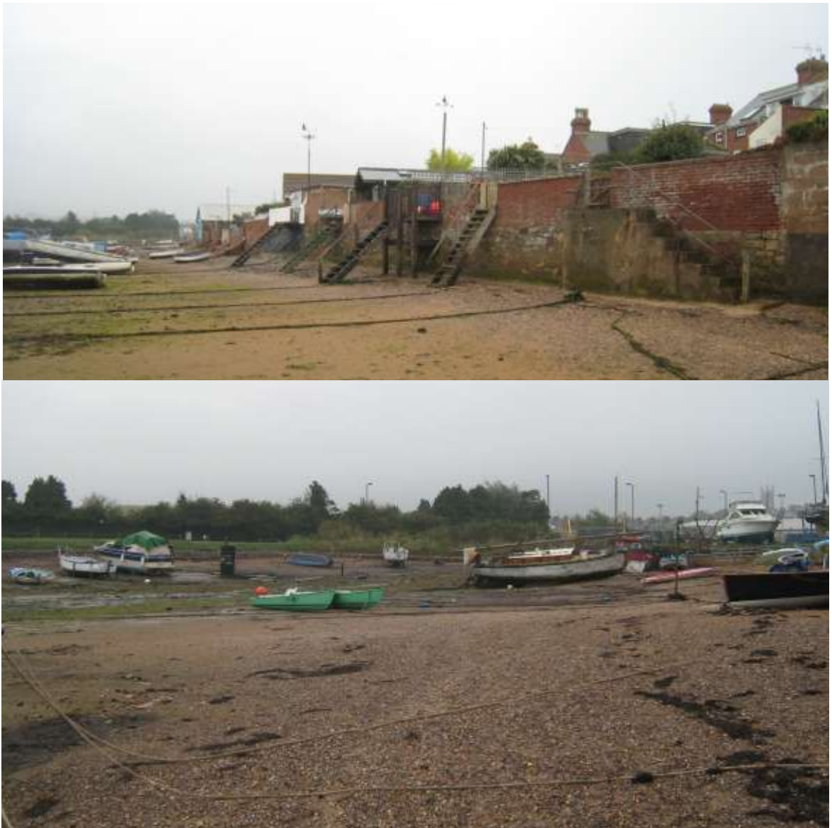
Figure 4.9 – Photographs of Camperdown Terrace, slipway and boatyard area.
