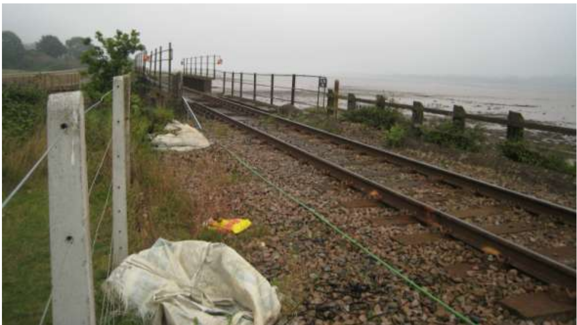
Figure 4.13 – Photograph of railway line at Exton.
