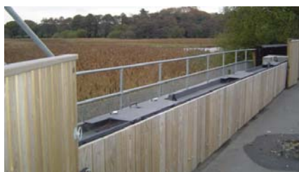
↑ Flood alleviation scheme at Lymington, completed in 2008.
