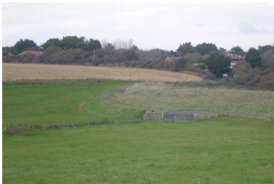
↑ Flood attenuation dam upstream of Milford-on-Sea.
