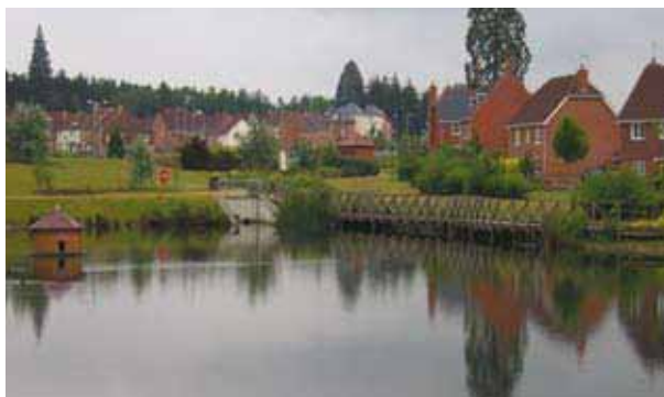
Elvetham Pond, part of the SUDS drainage scheme at a housing development in Fleet, Hampshire. Image courtesy of the Environment Agency.
