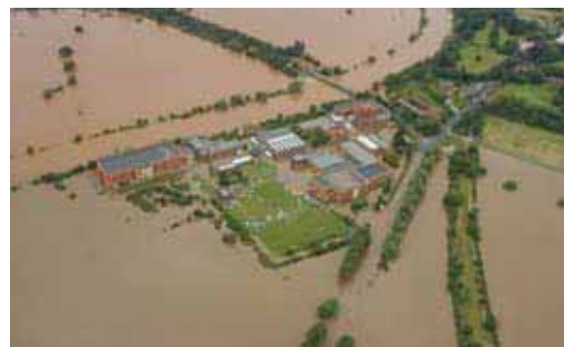
Flooding around Mythe Water Treatment Works, Gloucestershire. Image supplied courtesy of Severn Trent Water Limited.
