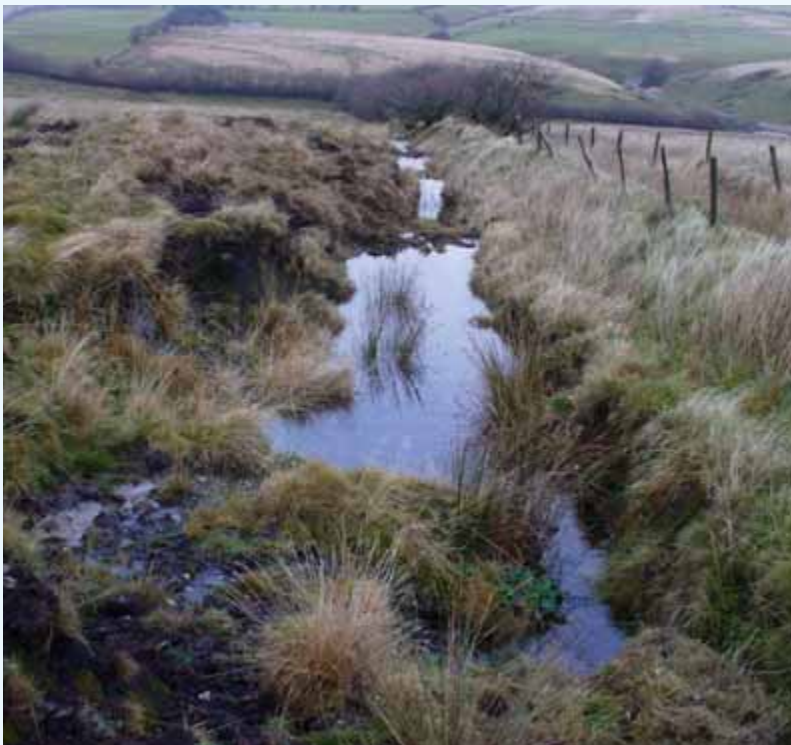
← Blocking ditches with peat dams to increase water storage.
