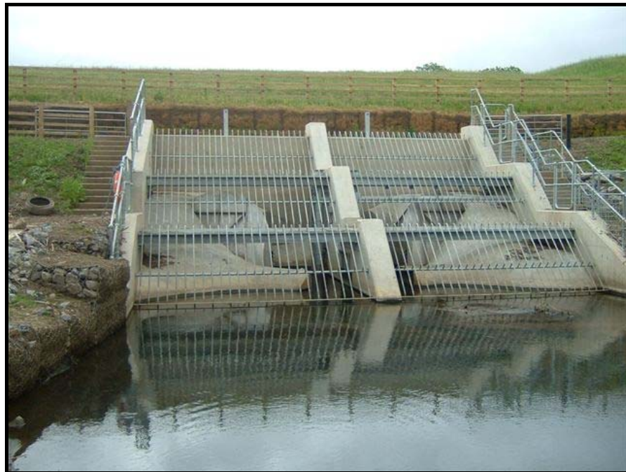
Photo 3: River Gaunless – Outlet structure with screen and flow controllers
