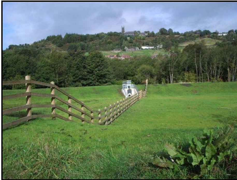
Photo 7: Millwood FSA - gated outlet
