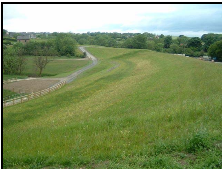
FSA Online Dam and Spillway
