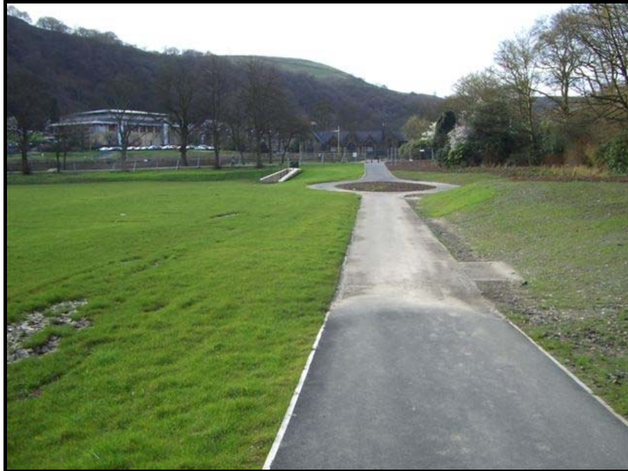
Photo 4: Centre Vale Park FSA and inlet structure
