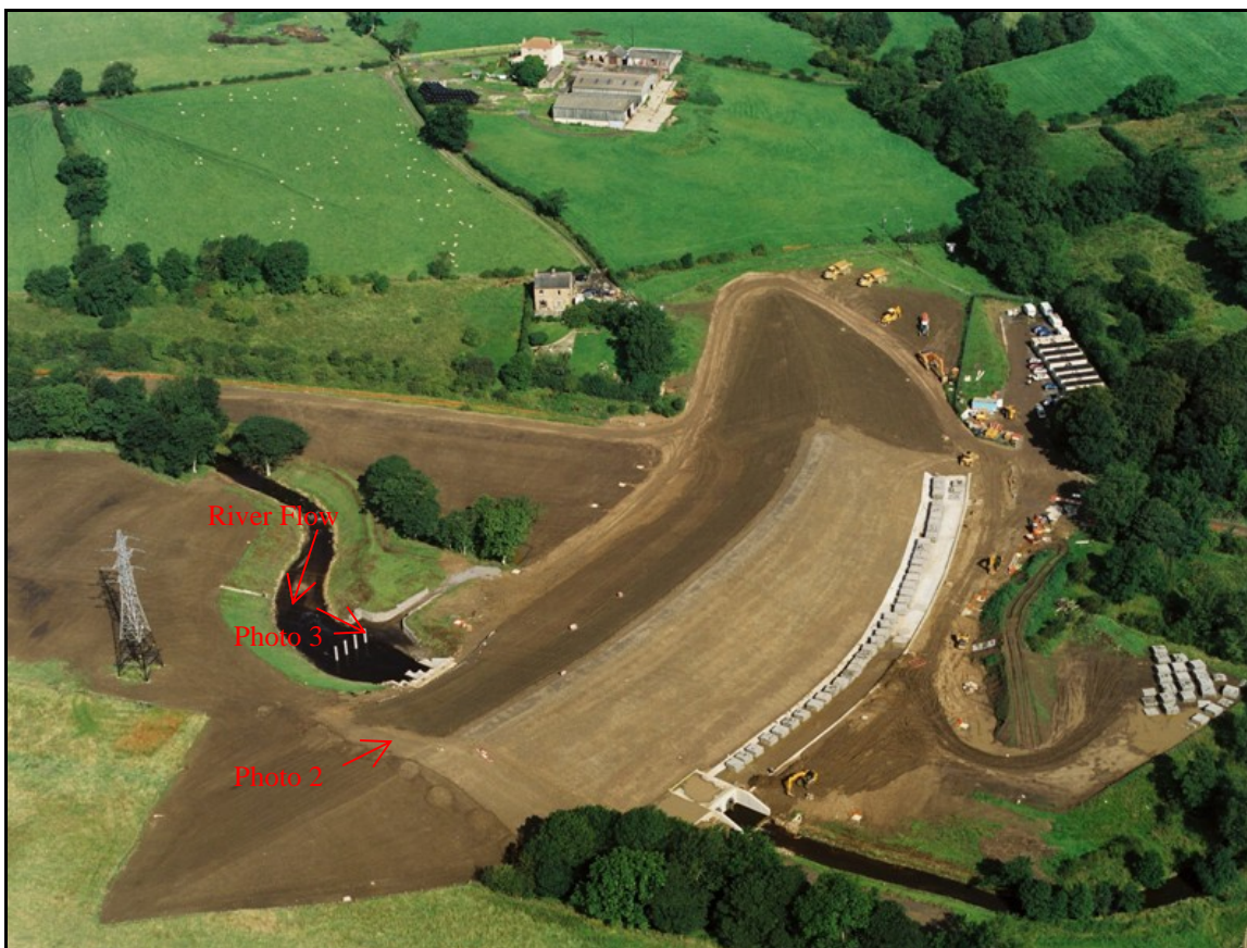
Photo 1: River Gaunless – Impounding FSA (at end of construction)
