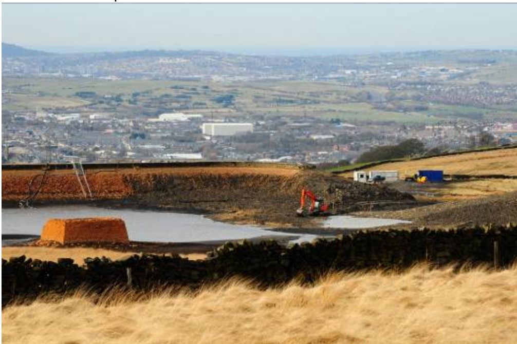
Figure 6.1 The 'notching-through' of Hameldon Reservoir
