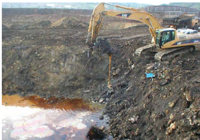
Photograph 1: Excavation and removal of contaminated soil (©Celtic Walters Land Ltd., 2005).
