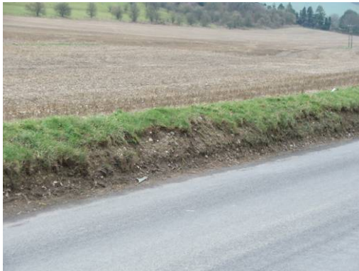
Eroding road banks upstream of Wylie river. Banks used to be four feet high – now degrading to two feet.
