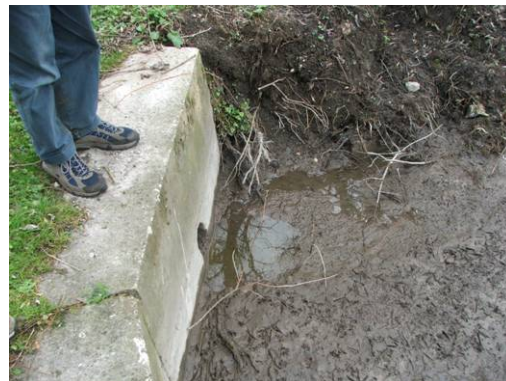
Sediment outflow directly below road – major problem, and needs frequent dredging to unblock road drain to prevent flooding of main A36.
