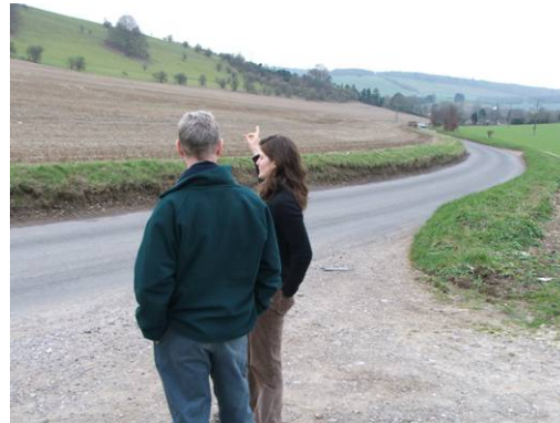
Eroding road banks upstream of Wylie river. Banks used to be four feet high – now degrading to two feet.
