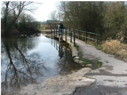
Widened river bed at ford
