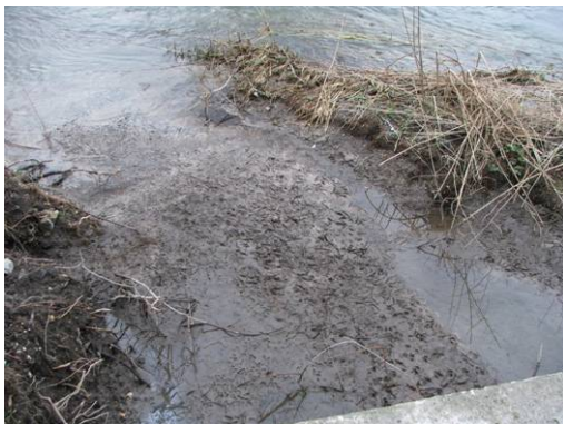
Sediment outflow directly below road – major problem, and needs frequent dredging to unblock road drain to prevent flooding of main A36.
