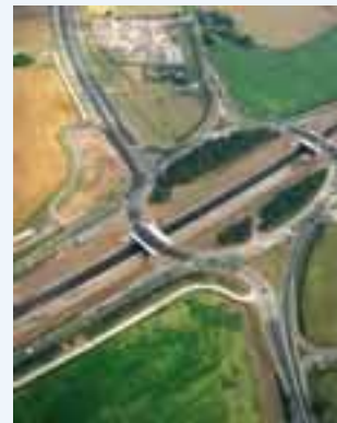
A5 Weeford - Fazeley improvement follows part of the Roman road Watling Street
