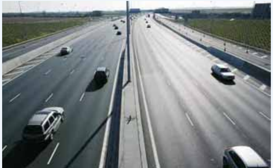
The new widened section of the M25
