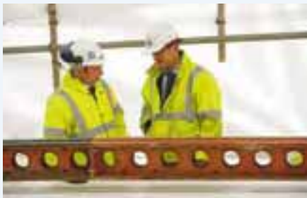
Fabrication of an innovative 'plastic bridge' on the M6 near junction 32
