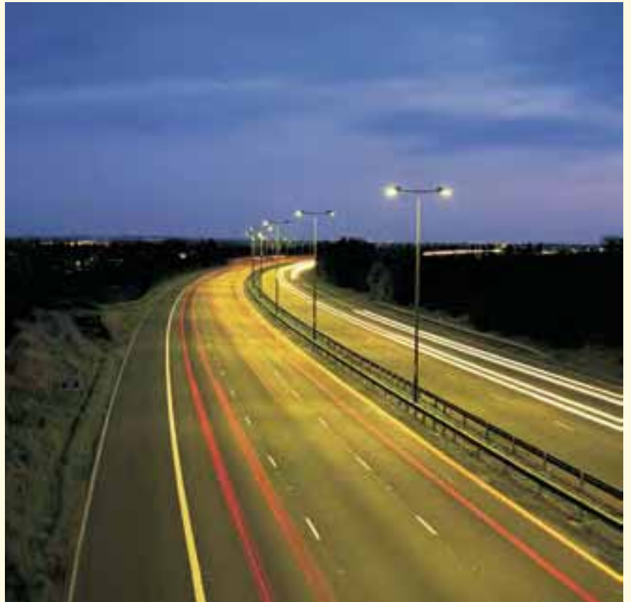
Environmentally friendly street lighting on the M1 Nottingham
