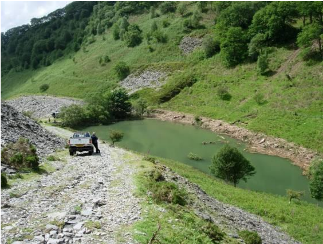
Figure 3.3 General view of the reservoir (Photo courtesy of Alan Warren)
