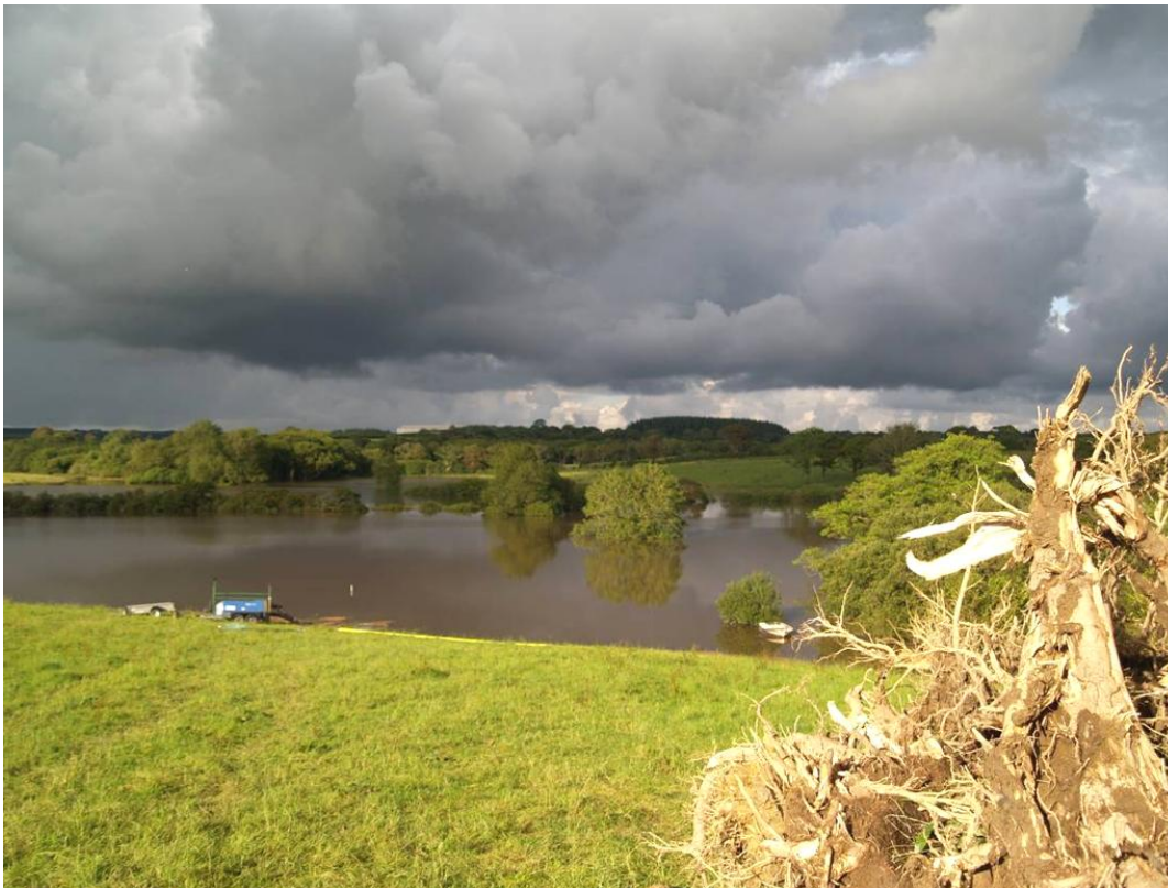
Figure 3.11 Impoundment against the canal embankment due to the collapse of the masonry culvert (Photo courtesy of David Harker)
