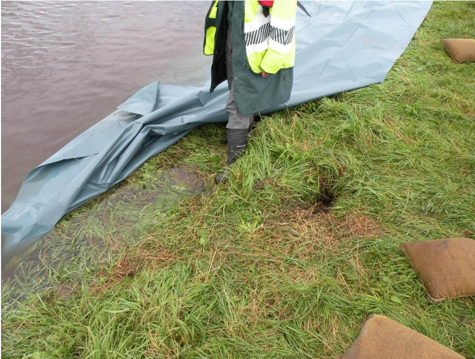
Figure 3.12 Animal holes on the crest of the river defence embankment (Photo courtesy of John Falkingham Associates)
