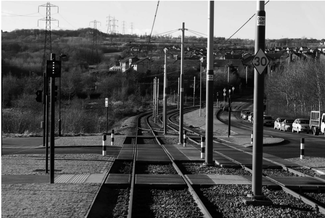
Pedestrian and highway crossings on the tramway in Sheffield, shown from the perspective of the tram driver. Note the tramway signals and ordinary traffic lights.
