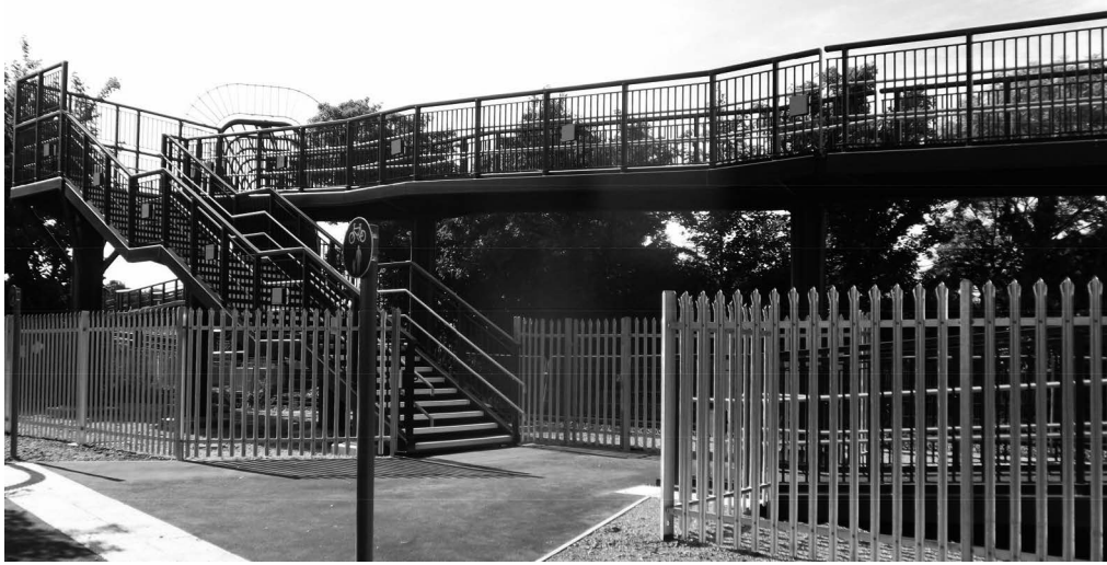
Footbridge at Fishbourne, East Sussex, built to provide a step-free replacement for the public footpath user-worked level crossing. The local authority and Network Rail are co-operating to seek permanent closure of the level crossing. Credit: Network Rail.
