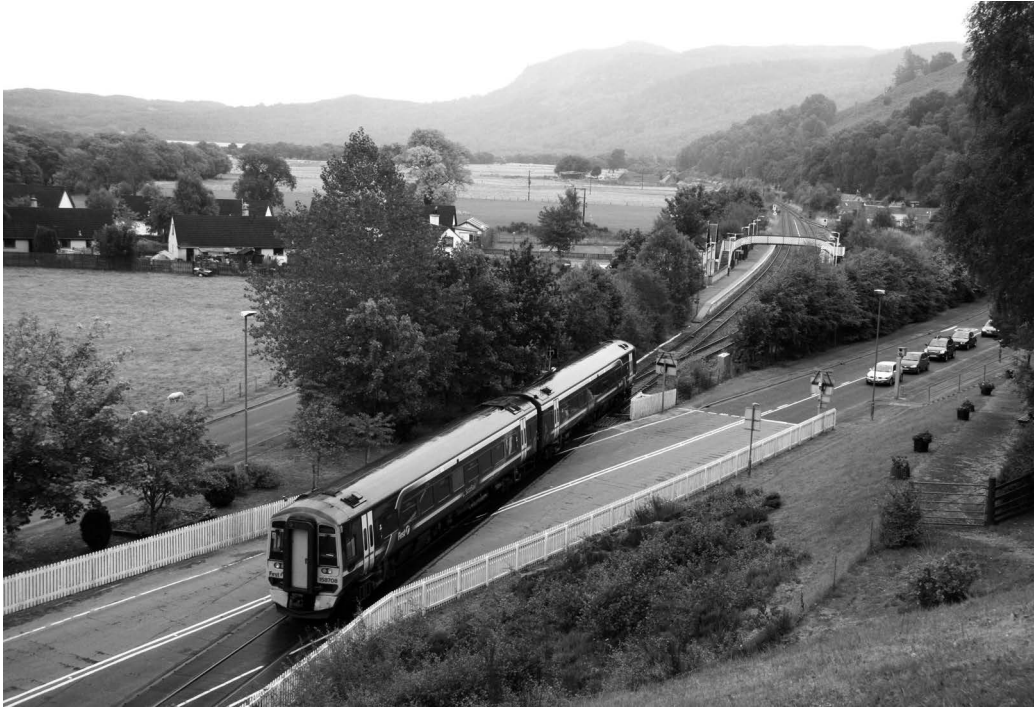
The automatic open (ungated) locally monitored level crossing (AOCL) at Garve Station on the Inverness to Kyle of Lochalsh line seen from the hillside. Credit: John Furnevel.
