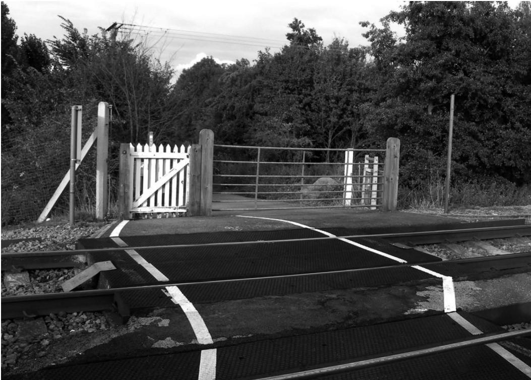
Gipsy Lane level crossing, Needham Market, Suffolk. The private road crossing has been closed by agreement between Network Rail and the beneficiary. The public footpath crossing remains in use. Credit: Rail Accident Investigation Branch.
