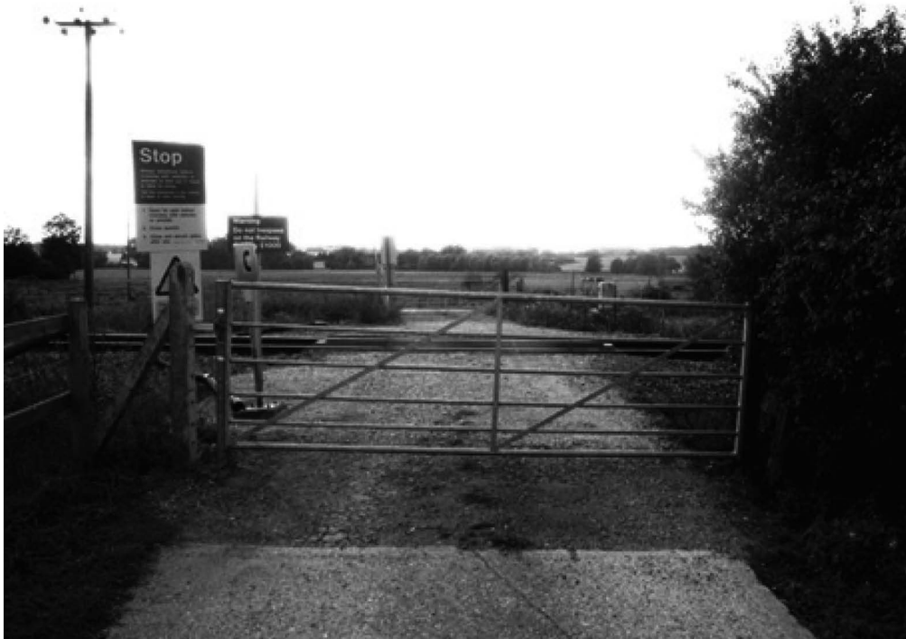
Sewage Works Lane level crossing, a user-worked, private level crossing near Sudbury, Suffolk. Credit: Rail Accident Investigation Branch
