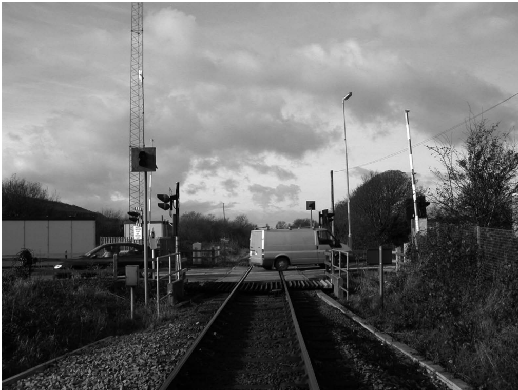
Llanbadarn automatic half-barrier level crossing (locally monitored), near Aberystwyth, seen from the train driver's perspective. Credit: Rail Accident Investigation Branch.
