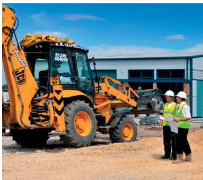
Picture: Construction at Coney Green Industrial Estate.
