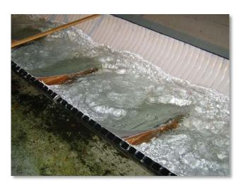
Culvert with baffles to improve eel passage
