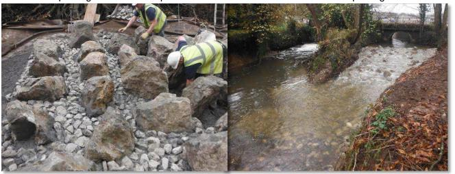
LEFT: Smaller rocks being placed by hand into the concrete surface of the rock ramp at Sharpsbridge. RIGHT: Completed rock ramp including downstream rock toe.
