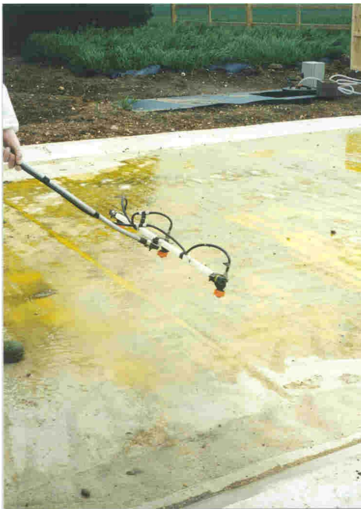
Figure 4.8: Application of washdown liquid mixture to concrete intercept using hand sprayer
