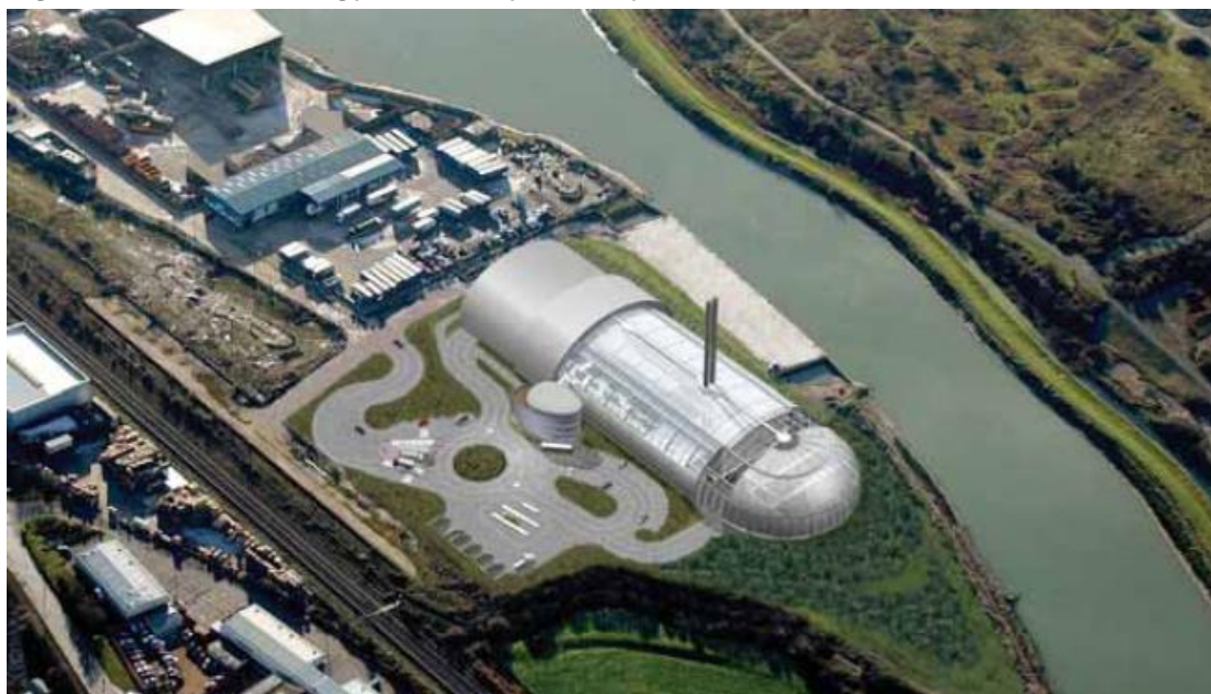
Figure 11 Veolia Energy Recovery Facility at Newhaven
