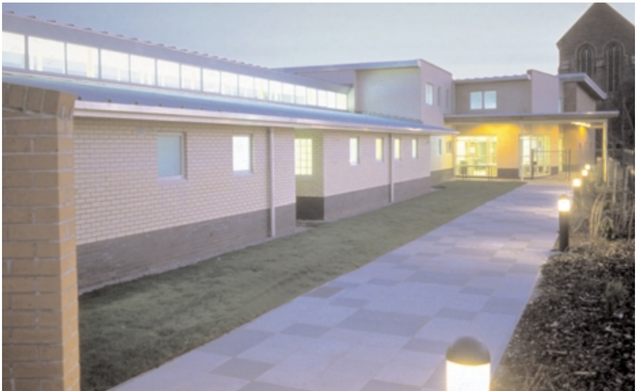
SMALL HEATH HEALTH CENTRE, NORTHERN BIRMINGHAM MENTAL HEALTH NHS TRUST: PHOTOGRAPH COURTESY MAAP
