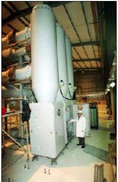
Figure A1-4: Indoor GIS circuit breaker
