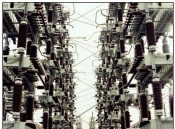
Figure A1-13: A Capacitive Reactive Compensator
