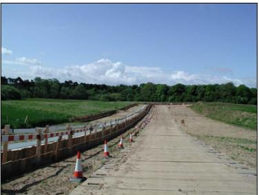
Figure A1-22: Access Swathe for Underground Cable Installation
