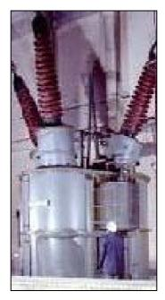
Figure A1-12: Inductive Reactive Compensator
