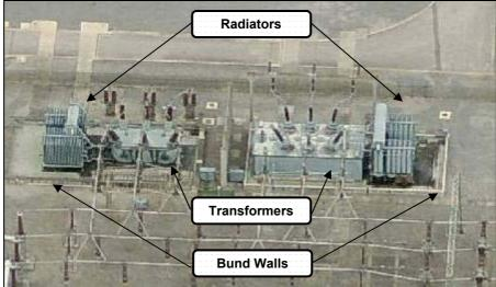
Figure A1-9: Typical 1100MVA Transformer Installation
