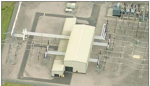
Figure A1-3: Aerial view of typical indoor, GIS substation
