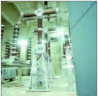
Figure A1-6: Indoor 275kV AIS circuit breaker
