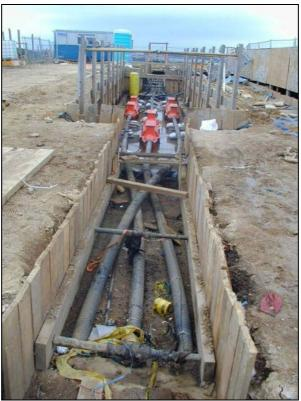
Figure A1-19: Underground Cable Joint Trench
