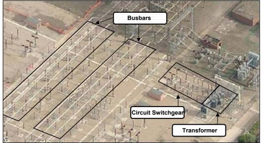
Figure A1-1: Busbars, Switchgear and Transformers
