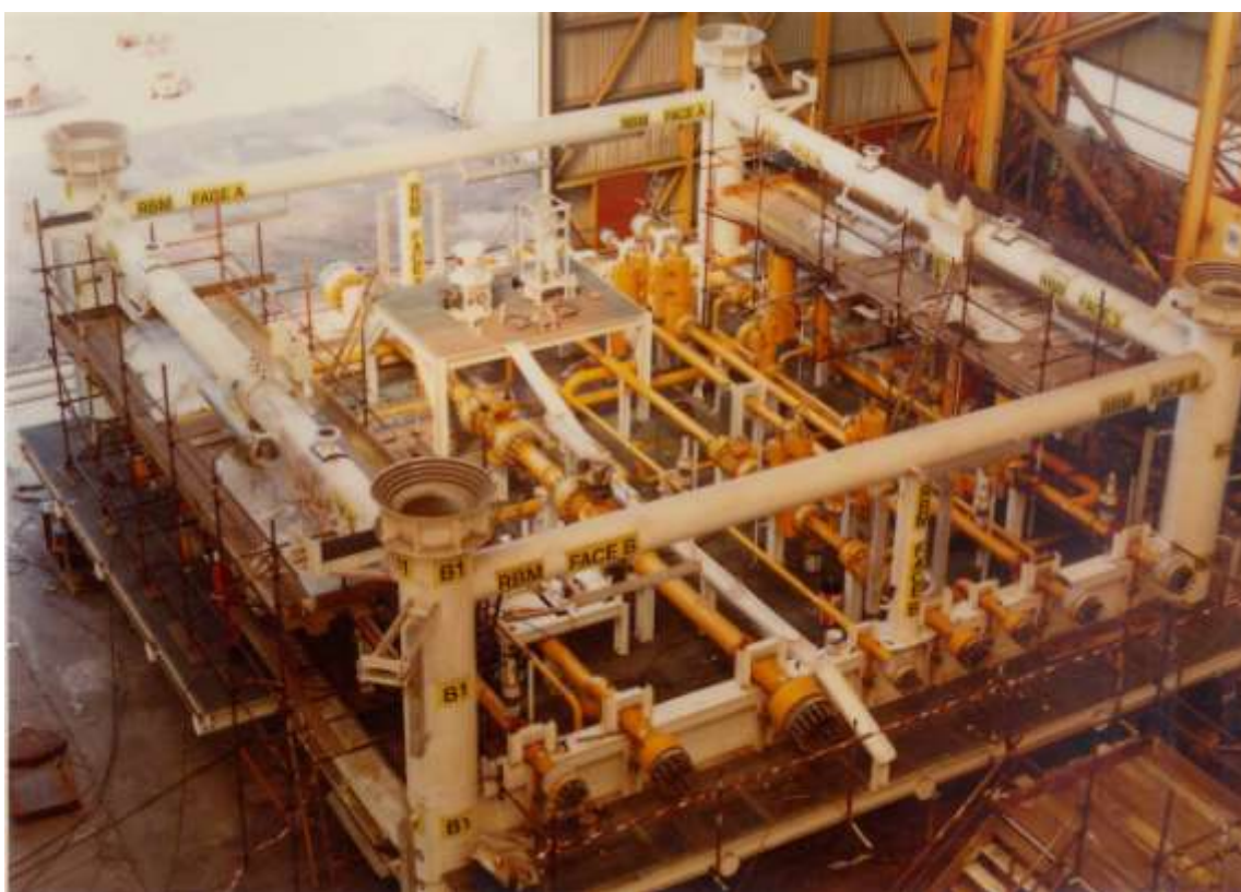
Figure 4.2: Riser Base Manifold (RBM)
