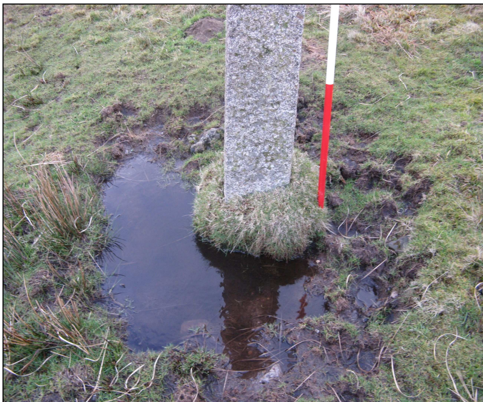
Fig 4 Boundary stone 1150912. Erosion hollow again active as a result of livestock using it as a rubbing post
