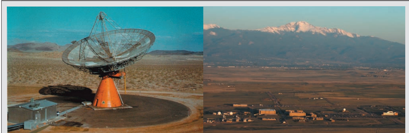
Illustration 1.39 – Ground Support Elements. Two aspects of the ground segment illustrated. The picture on the left shows an early satellite ground antenna installed at NASA/JPL’s Goldstone ground station in the Mojave Desert in California. This particular antenna was installed to support the Project ECHO passive communications experiment described in Chapter 3. The picture on the right shows Schriever AFB in Colorado. The Master Control Station for the Global Positioning System (GPS) constellation operates from here, alongside other military space capability. (Images courtesy of NASA/JPL (left) and USAF (right))
