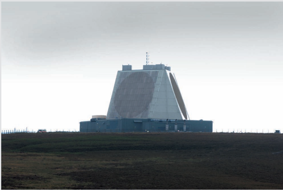
Illustration 4.7 – The UK Contribution to Missile Warning and Space Surveillance. RAF Fylingdales on the North Yorkshire Moors houses a Raytheon Solid-state Phased Array radar (SSPAR), which in conjunction with other similar sites elsewhere contributes to Allied missile-warning and space-surveillance roles. The SSPAR replaced a mechanically-scanned radar installation in 2000, housed in formerly well-known ‘golfball’ radomes. The RAF Fylingdales installation is unique in the Allied radar chain in having a 360° field of view, provided by the 3 faces of the antenna. (Crown copyright photograph).
