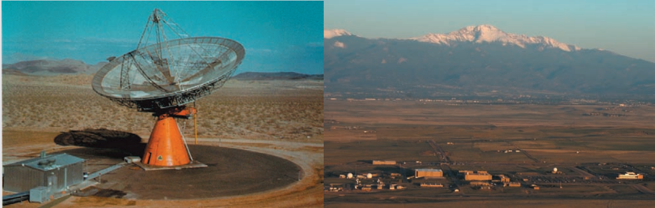
Illustration 1.39 – Ground Support Elements. Two aspects of the ground segment illustrated. The picture on the left shows an early satellite ground antenna installed at NASA/JPL's Goldstone ground station in the Mojave Desert in California. This particular antenna was installed to support the Project ECHO passive communications experiment described in Chapter 3. The picture on the right shows Schriever AFB in Colorado. The Master Control Station for the Global Positioning System (GPS) constellation operates from here, alongside other military space capability. (Images courtesy of NASA/JPL (left) and USAF (right))
