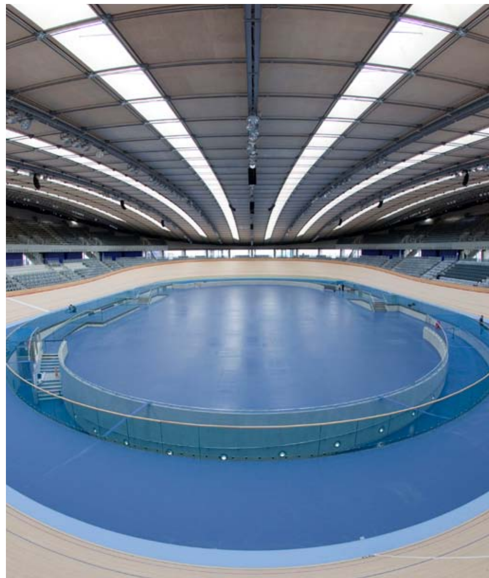
Velodrome – Built with 100% legally and sustainably sourced timber and is almost 100% naturally ventilated.
