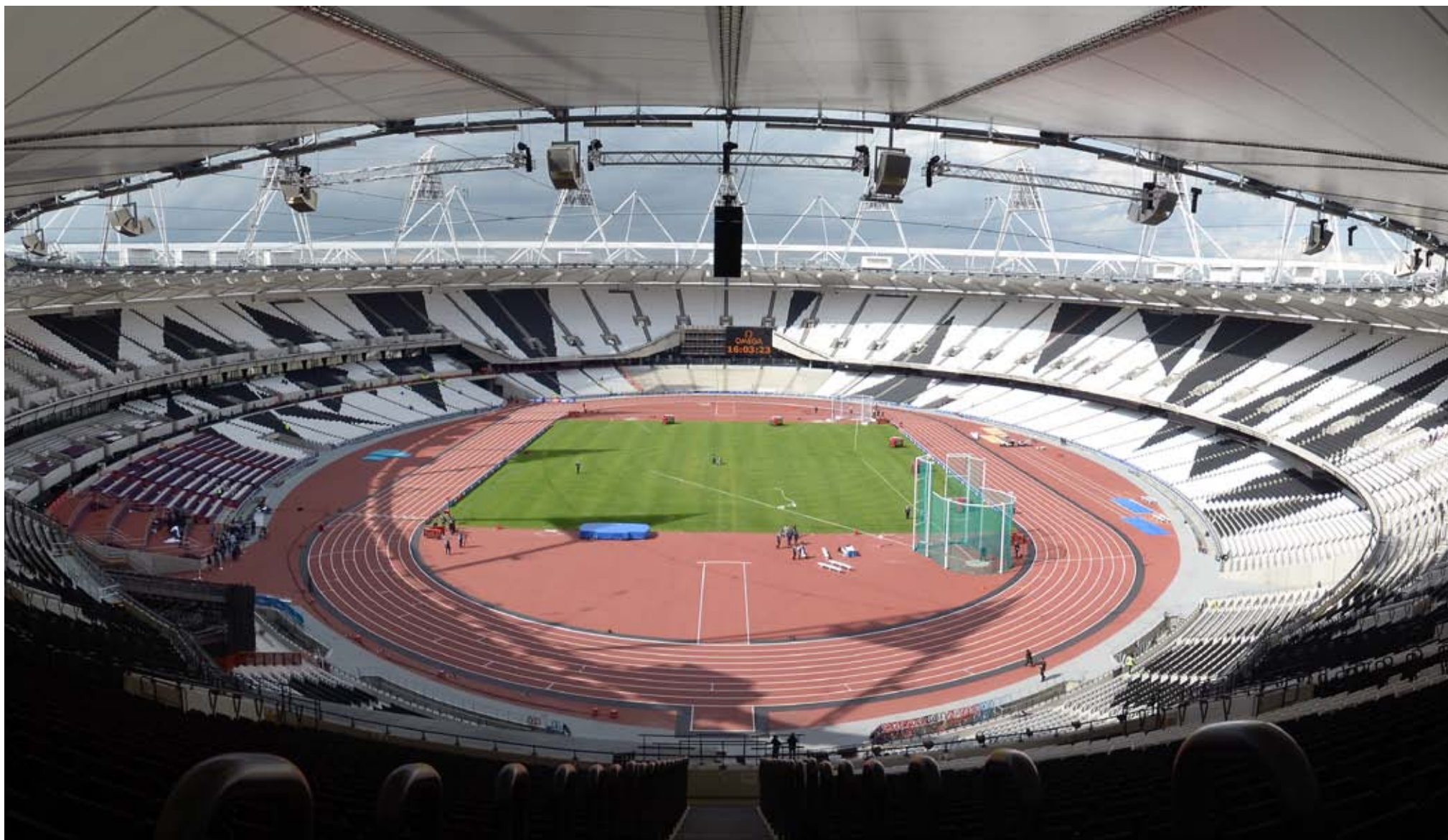
Olympic Stadium – The lightest Olympic Stadium ever built, containing just 10,000 tonnes of steel.
