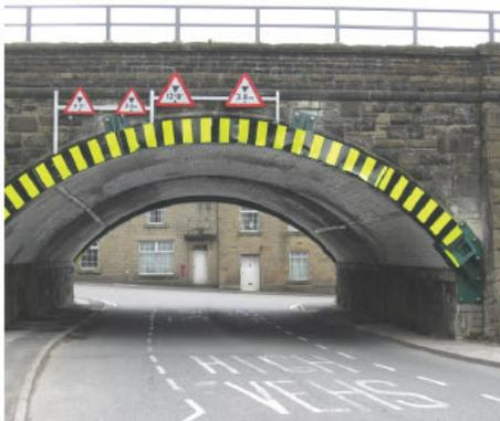
White lines on the road and 'goal posts' on the arch indicating the extent of the signed vehicle height limit
