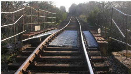
*Track distortion due to a bridge strike*
