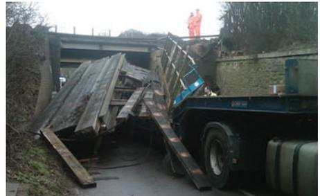
*Bridge dislodged from abutments onto the vehicle which struck it*
