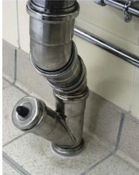
Where walk-in refrigeration and air-cooling plant is installed, drainage will need to be provided to accept the defrost condensate.
