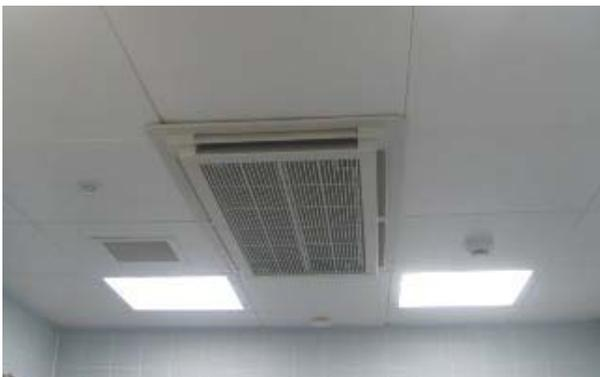
The cooling system shall be a ceiling mounted cassette unit of an adequate size to maintain the desired room temperature, be draught free, easy to clean and incorporate a bactericidal filter. Drainage may be required to receive condensate from the equipment.
