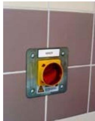
Combination ovens shall be fitted with interlocking isolation switches to prevent disconnection of the unit without prior isolation.
