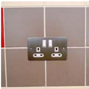
Sockets and switches shall be flush mounted and manufactured of impact resistant fascias, preferably of stainless steel; 'domestic type' plastic fascia plates are not acceptable. Sockets shall be provided for each item of equipment listed in the catering equipment schedule and located at a height suitable for the item of equipment. Mid-height sockets and switches, etc, shall be positioned in the centre of the colour banding centred on the centre of four tiles as illustrated.
