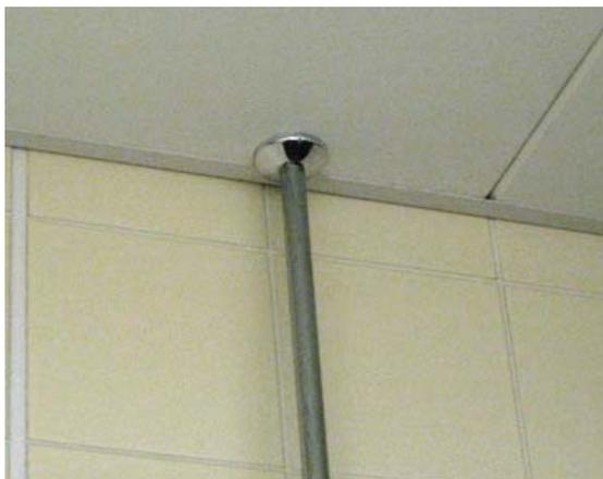
Pipe penetrations into walls and ceilings shall be fully caulked with mastic or grout as appropriate and fitted with cloaking rings or roses. (The fitting of cloaking rings and roses over unsealed penetrations is not acceptable)
