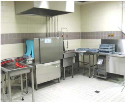
Adequate dedicated ventilation and extraction shall be provided to ensure that steam emitted from the utensil washing machine or steriliser sink does not give rise to condensation within the room.
