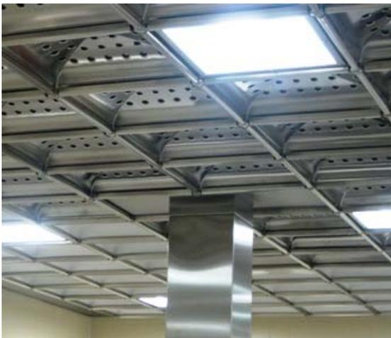
The system shall be designed to provide a modular ceiling system with facilities for 85% minimum grease extraction, make up air and lighting. Sealed, integrated lighting units shall be incorporated, and installed in sufficient number and distributed to provide an overall 500 lux at work surface height without shadows.
