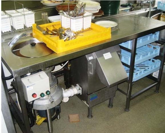
processed through maceration from where it is passed through a de-waterer that extracts up to 80% of the liquid from the macerated food mass. The liquid goes direct to drain as above, and the solids are collected for direct disposal to the refuse collection system. The solid food waste requires additional processing either by double bagging for forwarding to the refuse skips for subsequent collection by the appointed waste contractor, or further on site processing.
