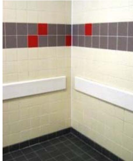
Tiles shall have a plain, smooth surface to allow ease of cleaning and lay flush with the floor coving to the ceiling without the inclusion of projections or ornamentation. (See 7.2)
