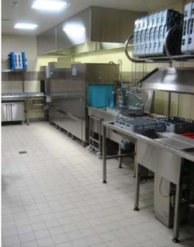
Where staff use trolleys to clear the tables, the crockery wash should cater for the receiving of loaded trolleys by provision of a parking space adjacent to the unloading/scraping area.
