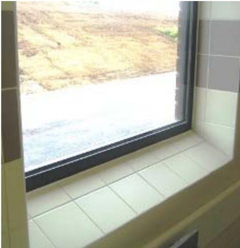
In all catering areas including the utensil and crockwash, serveries and pantries, windows shall be sealed and do not, therefore, require a fly screen to be fitted. Where opening windows are provided, fly screens shall be fitted as required by the EHO. Fly screens shall be of robust construction and capable of being easily removed and fitted for cleaning and maintenance purposes.
