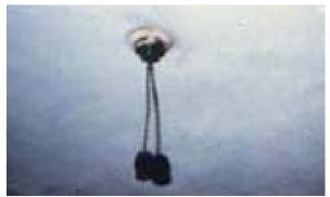
Original cloth covered wiring and pin sockets: from a house built in the 1920s.
