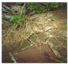
Risk from falls on the level: broken and uneven paving.
