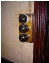
**Fire hazard – old wiring:** increases the risk of a fire starting (and electrocution).
