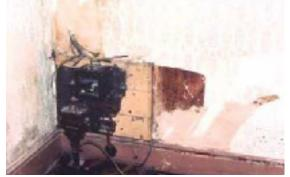
Old wiring and sockets: a number of which look damaged.
