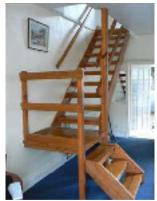
**Risk of falls between levels:** large gaps in balustrade and insufficient area of platform part way up.
