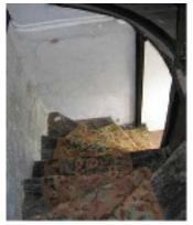
**Risk from fall on the stairs:** steep, narrow winding with no handrail.
