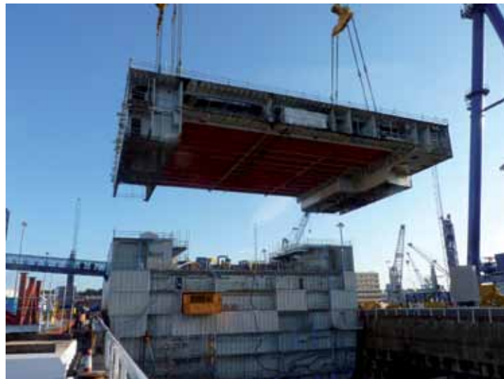
The first centre block is lifted into place at by the Goliath crane at Rosyth
