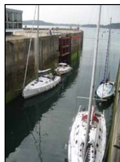
Plate 4.2 Small craft lock at La Rance Tidal Power Barrage
