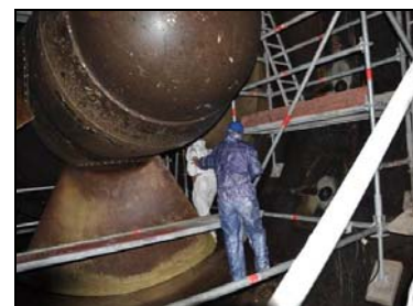
Plate 4.3 Bulb turbine at La Rance Tidal Power Barrage (10MW with 5.7m diameter)
