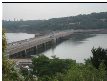
Plate 4.1 La Rance Tidal Power Barrage (750m long with 24 bulb turbines)
