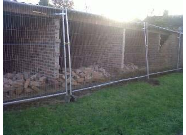
Demolition of garages
