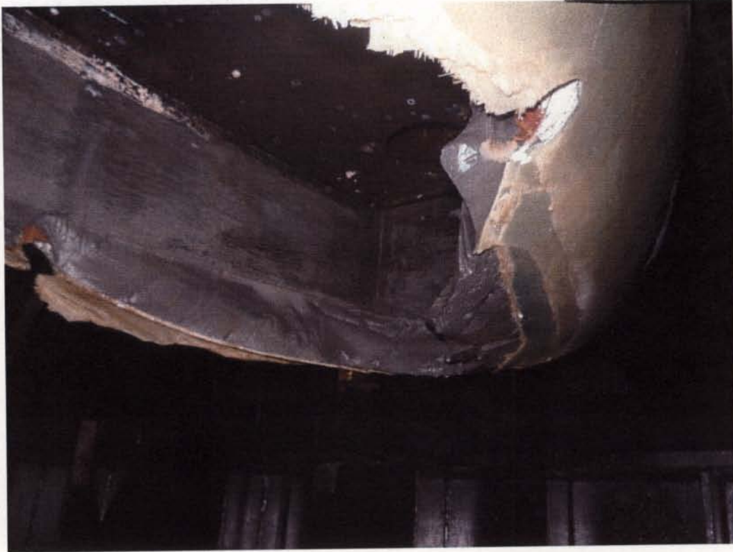
Figure 8 – Internal Damage to GRP Rudder Skeg.
