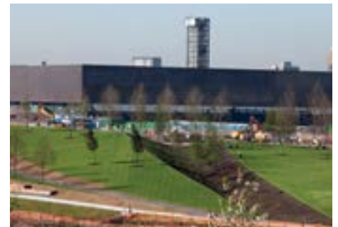
The Park's new energy infrastructure will reduce carbon emissions
