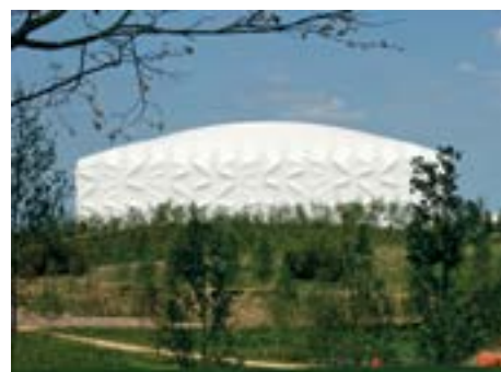
The Basketball Arena took just 15 months to build
