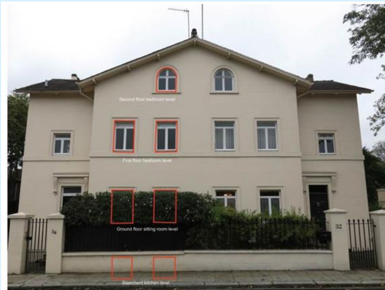
Figure 8: A view of 34 Park Village East. Windows where internal secondary glazing will be installed are annotated in red.
