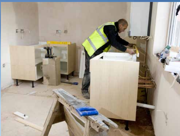
Upgrades underway on Service family homes at High Wycombe
