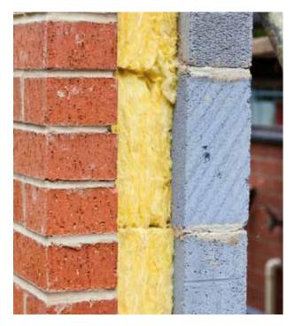
1.31 Houses built since 1900 usually have a cavity wall, this can be filled with insulating foam that effectively traps heat inside the building. Modern houses are built with pre-filled cavities so no retrofit is necessary, but in older houses insulating a cavity can reduce heat loss by around 20%.
