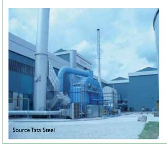
Once the Oxidiser is at operating temperature it requires no additional fuel. A secondary heat exchanger routes waste heat back to the process ovens, reducing the amount of natural gas required. In addition, supplementary fuel injection has been installed, for greater efficiency.
