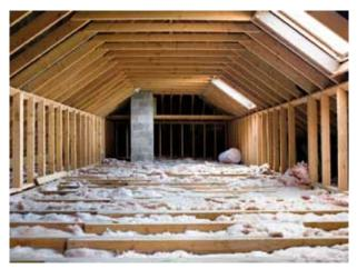
1.28 Loft insulation reduces heat loss from a building by up to 27% and is usually straightforward to install. A DIY installation can cost as little as £25, and professional installers typically charge around £300.
