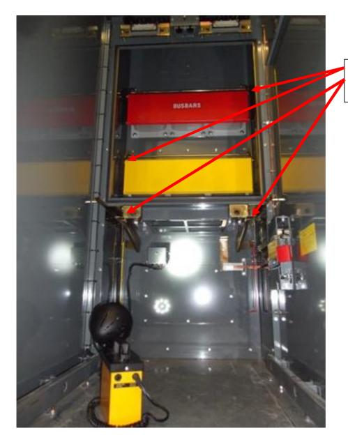
Split pins located here require checking to make sure legs are bent fully.
