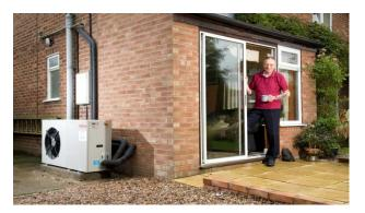
ASHPs are relatively simple and easy to install, with little routine maintenance needed generally. They perform best in warmer weather. Issues that need to be taken into account when installing ASHPs are potential noise and planning consent implications.
