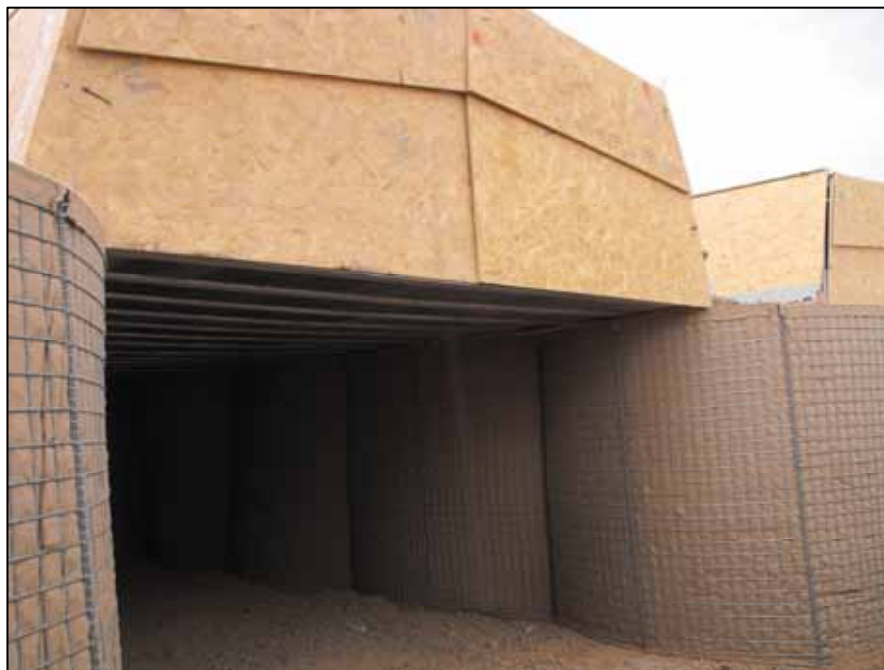
Figure 3.6 – Lightweight Bunker Roof
