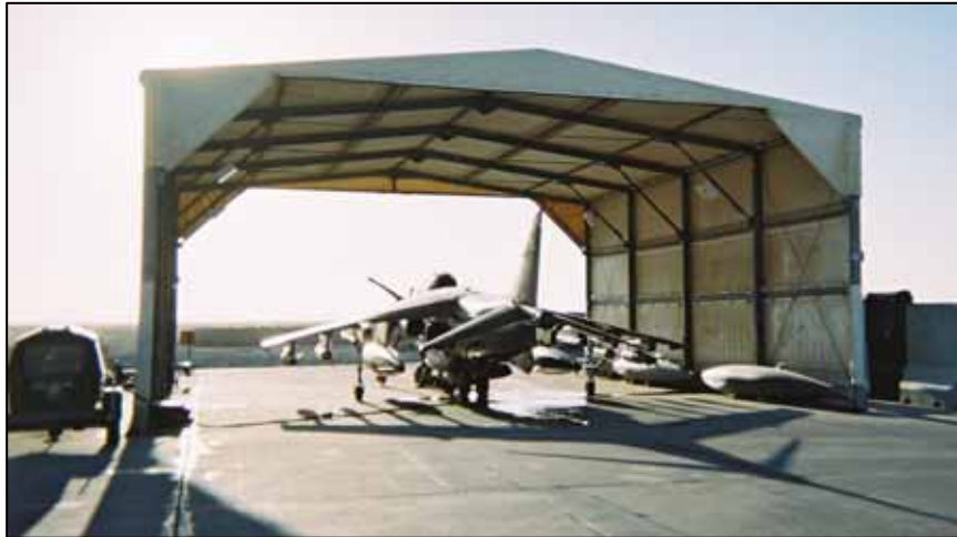
Figure 5.6 – Rapid Erect Building
