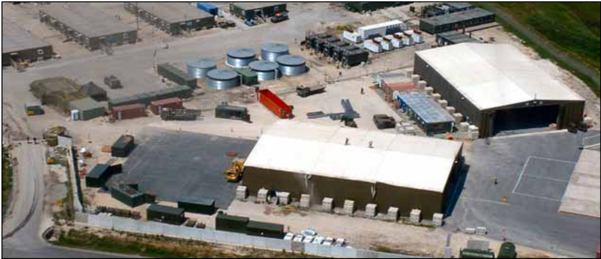
Figure 5.5 – Rapid Erect Hangar
