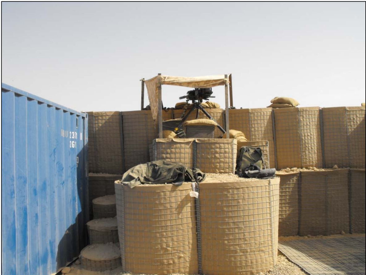
Figure 3.1 – Hesco Bastion walls
