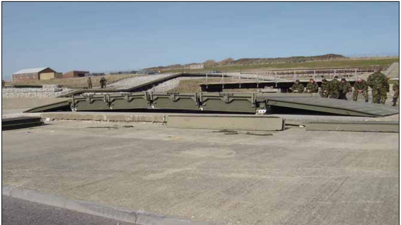
Figure 2.2 – Medium Girder Over Bridge
