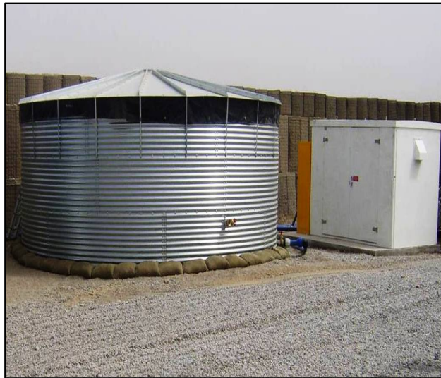
Figure 7.3 – Borehole Well-head Unit
