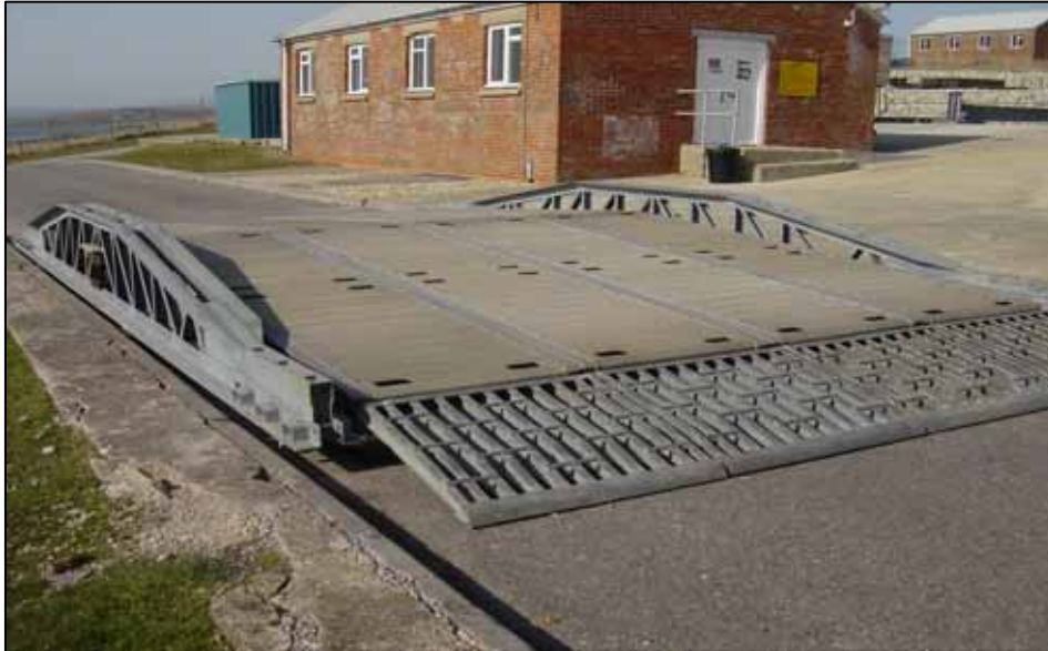
Figure 2.3 – Heavy Girder Over-bridge
