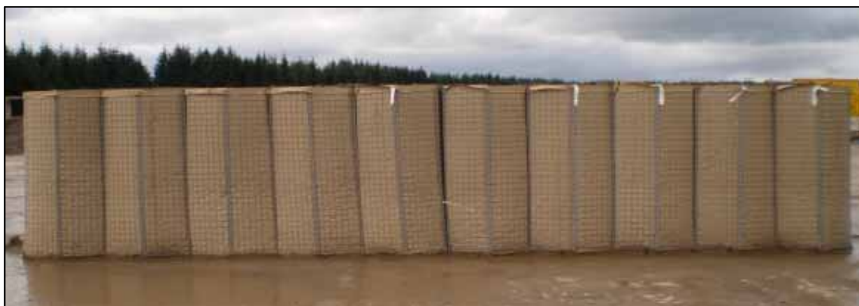
Figure 3.2 – Enhanced Protective Wall
