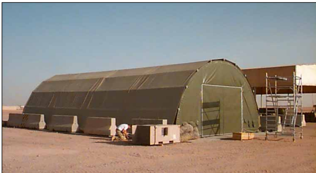
Figure 5.3 – Environmentally Controlled Ammunition Storage Shelter
