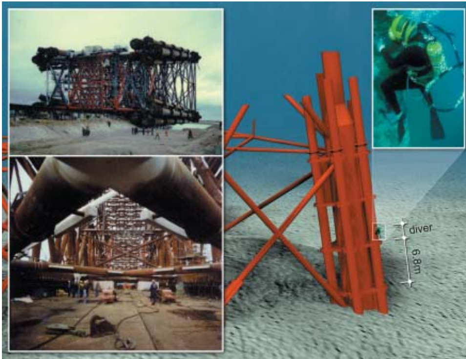
Figure 8.8: Computer generated diagram and photographs showing size and complexity of the bottle legs
