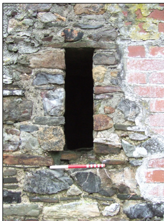
Fig. 67 – slit window of Bullock House. Scale: 30cm (TG)
