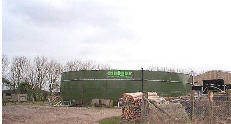
Plate 2. Above ground 'tin tank' slurry store.
