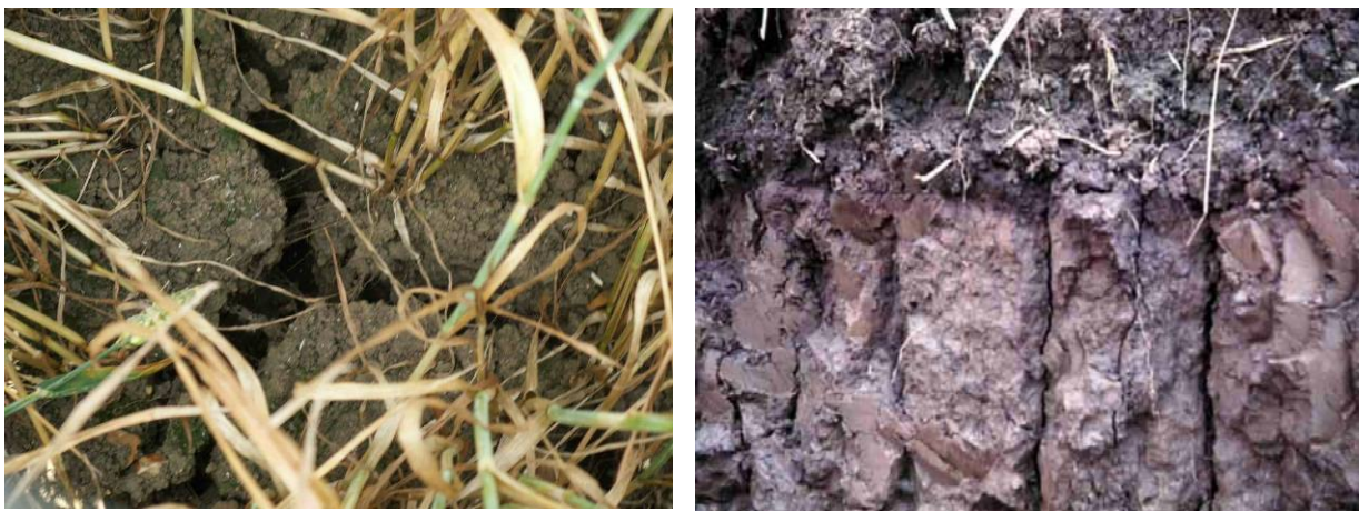
Plate 1. Cracks and fissures in clay soils.
